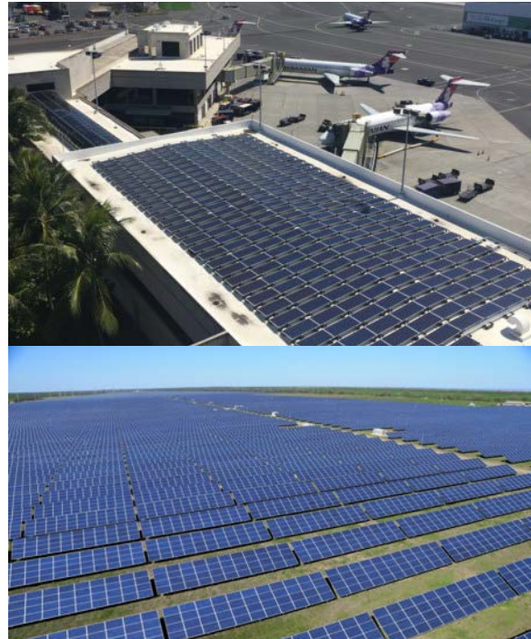
Figure 3: Examples of large roof-mounted and ground-mounted solar PV arrays.
