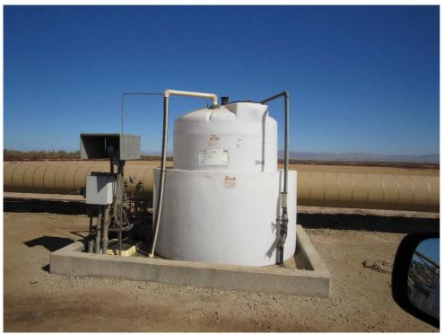
Photo 78: Looking GEO906 geothermal treatment liquid container located at the well pad.
