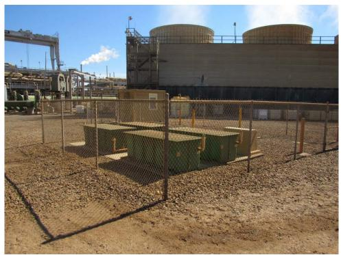
Photo 62: Looking at the waste treatment system are at the northwest corner of the cooling tower. The effluent from the waste treatment system gets reinjected with the brine into the reinjection wells.
