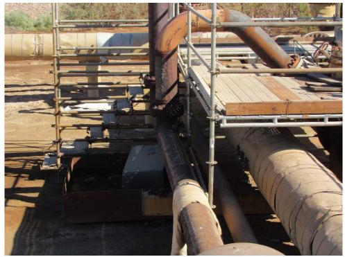
Photo 73: Looking at a secondary containment bin located under the vales at the pipe crossing road.
