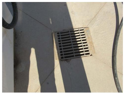
Photo 37: Looking at the drain within the fuel tank secondary containment area, this sump drains to the brine pond.
