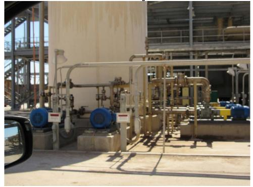
Photo 63: Looking at multiple pumps that are typical within the geothermal power plant and within a secondary containment berm.
