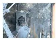
A content fire in the garage of this residence destroyed the PV inverter box.
