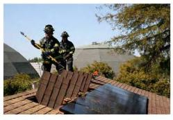
Firefighters need to practice and train for roof operations and ventilation techniques when photovoltaic systems are present
