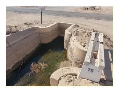
Figure 7: Overview of Spruce No. 3 Lateral, showing construction dates of 1956 and 1963, facing west/southwest. Located at the southeast corner of Hovley Road and Andre Road.
