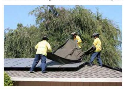
Fire departments should test their salvage covers on a PV array in advance of an incident to determine if they will successfully block light transmission.
