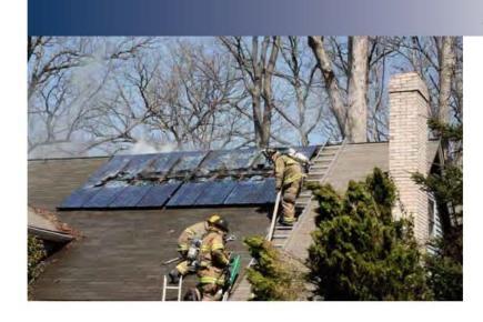
A roofing system, with two layers of composite shingles and a PV array may be compromised when affected by fire.
