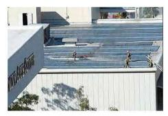
The modules on fire at the Long Beach Convention Center were damaged in shipping and field repaired by the manufacturer's rep prior to installation.
