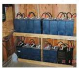
As with any utility supplied electrical source, an effort should be made to disconnect, or shut off the electrical current. Disconnect switches for PV systems equipped with batteries can usually be located near the battery bank and on the conductor(s) leading away from the batteries.
