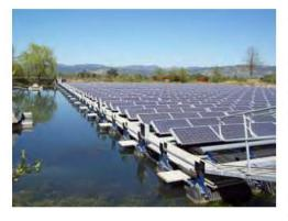
Float-o-voltaics (floating PV systems). Built on pontoons, these PV modules are mounted on a floating platform. They are likely to be found where there is a high land value, such as farm lands and there is a body of water nearby. At least two systems are currently in operation in California.
