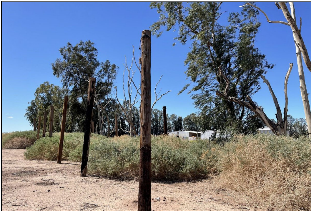
PHOTOGRAPH 6 Overview of Shade Structure Support Poles, Looking Southwest
