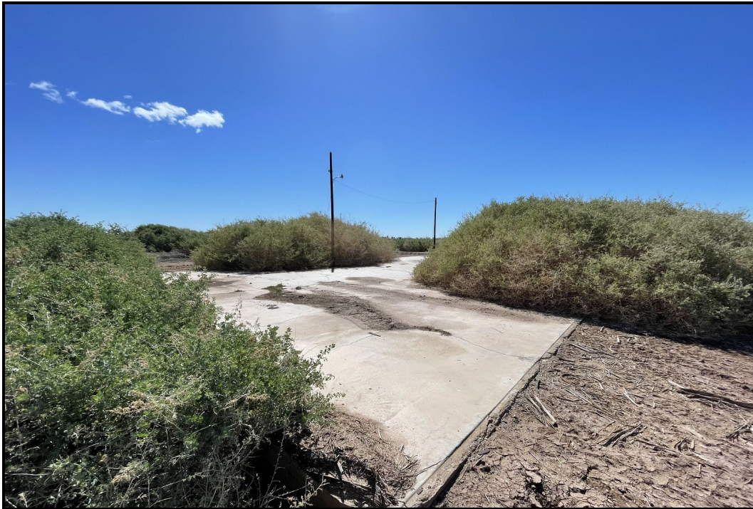
PHOTOGRAPH 5 Overview of circa 1980 Concrete Foundation in Southeast Project APE, Looking Southeast
