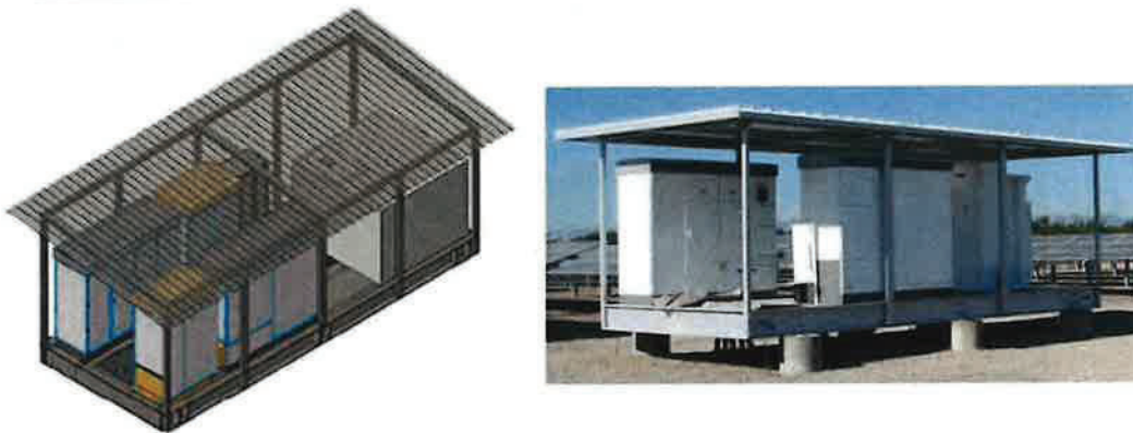
Typical inverter stations
