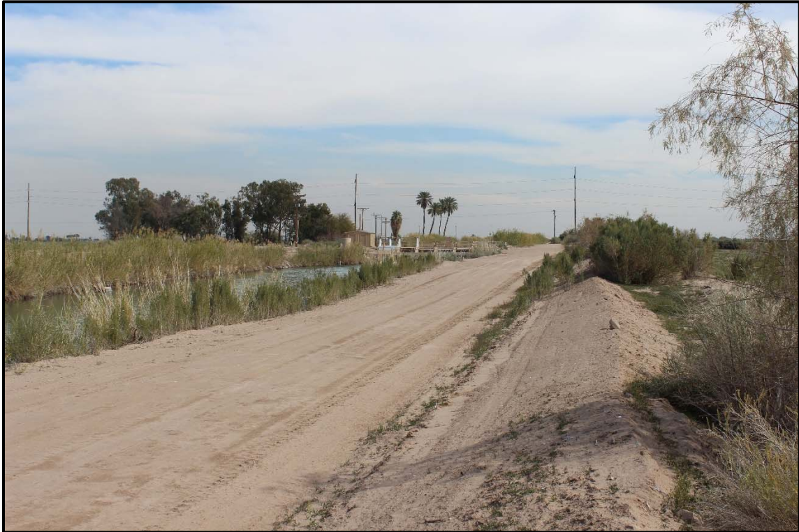
Photo 11: Westside Main Canal and Fern Heading on north boundary of subject property.
