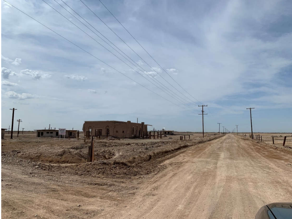
Photo 27: Looking south to southeast at the north end of the Gen-Tie line route on the east side of Davis Road.
