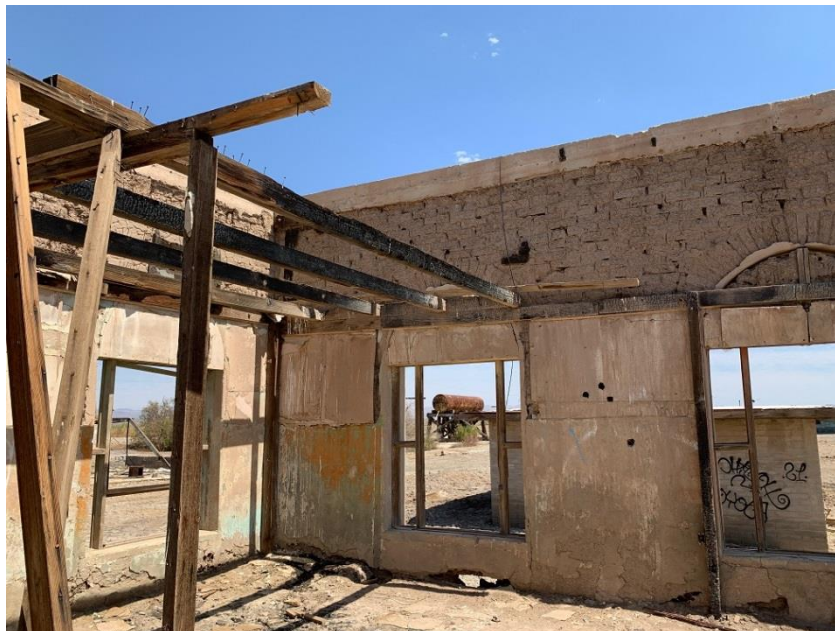
Photograph 2 – Example of multiple construction methods applied to preexisting structure.
