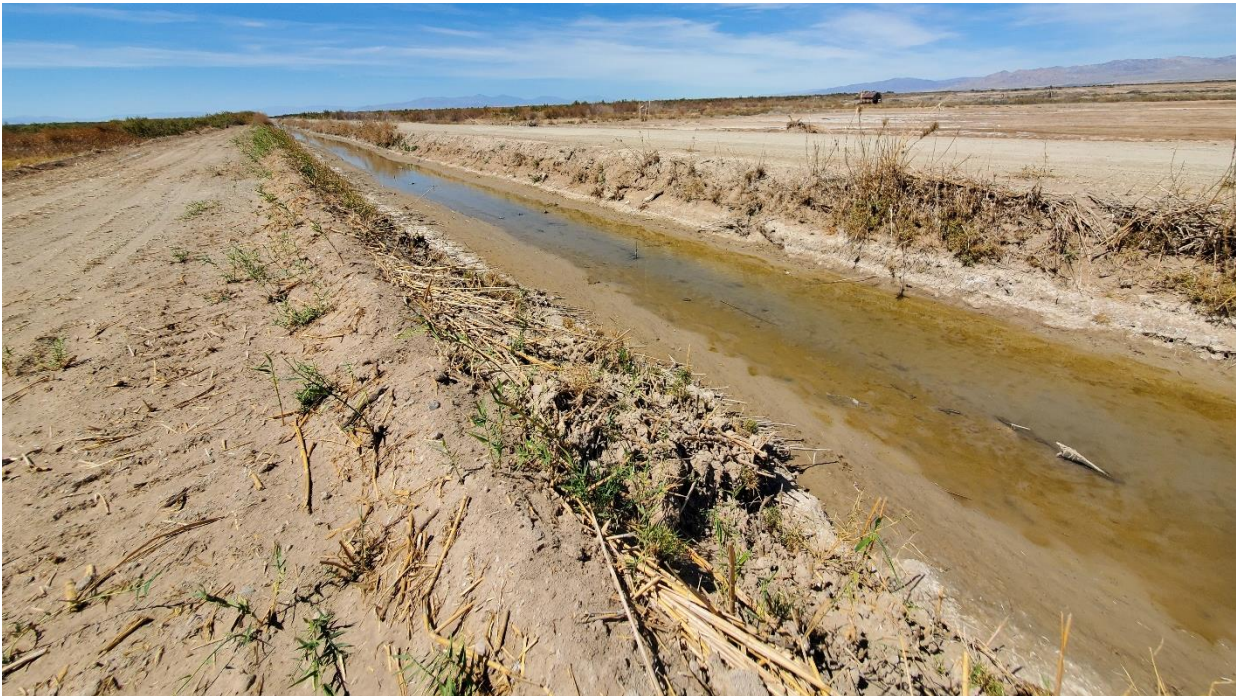
Photo 18: S-Drain at Davis Road.
