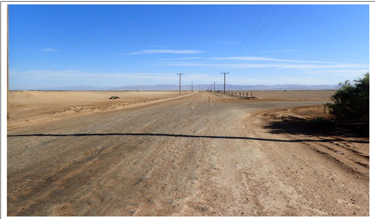
10. Davis Road looking north from McDonald Road: not BUOW foraging or burrowing habitat
