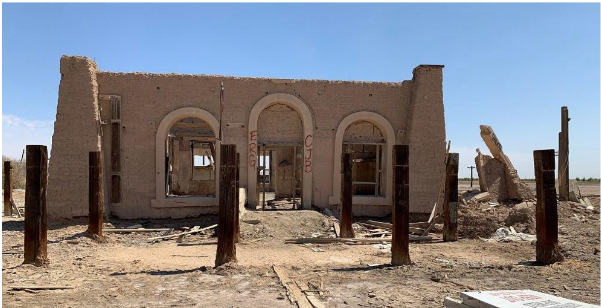
Photograph 5. TES-HK-001H: Street-side, western façade.
