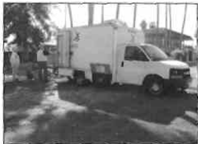
Video inspection operations at MH 26. Note the location of the manhole and sewer line at the rear of the van within private backyards; this is one of the more accessible locations.
