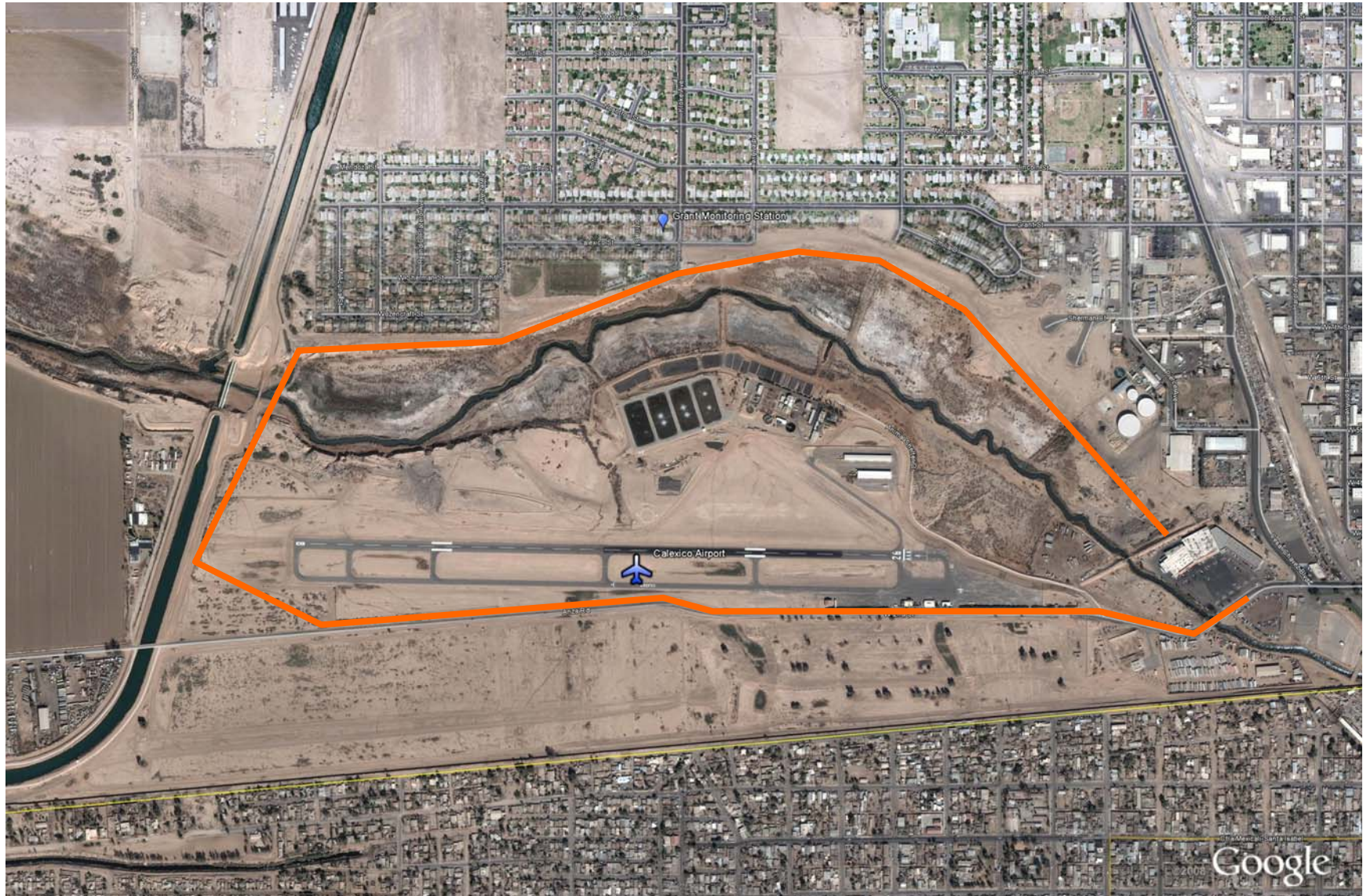
Figure V.B.1 Satellite image showing an enlarged view of the area directly south of the Calexico Grant station. The airport is fenced in within the boundaries delineated by the orange line.
