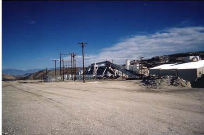
Overview of Quarry and Associated Facilities Facing Northeast
