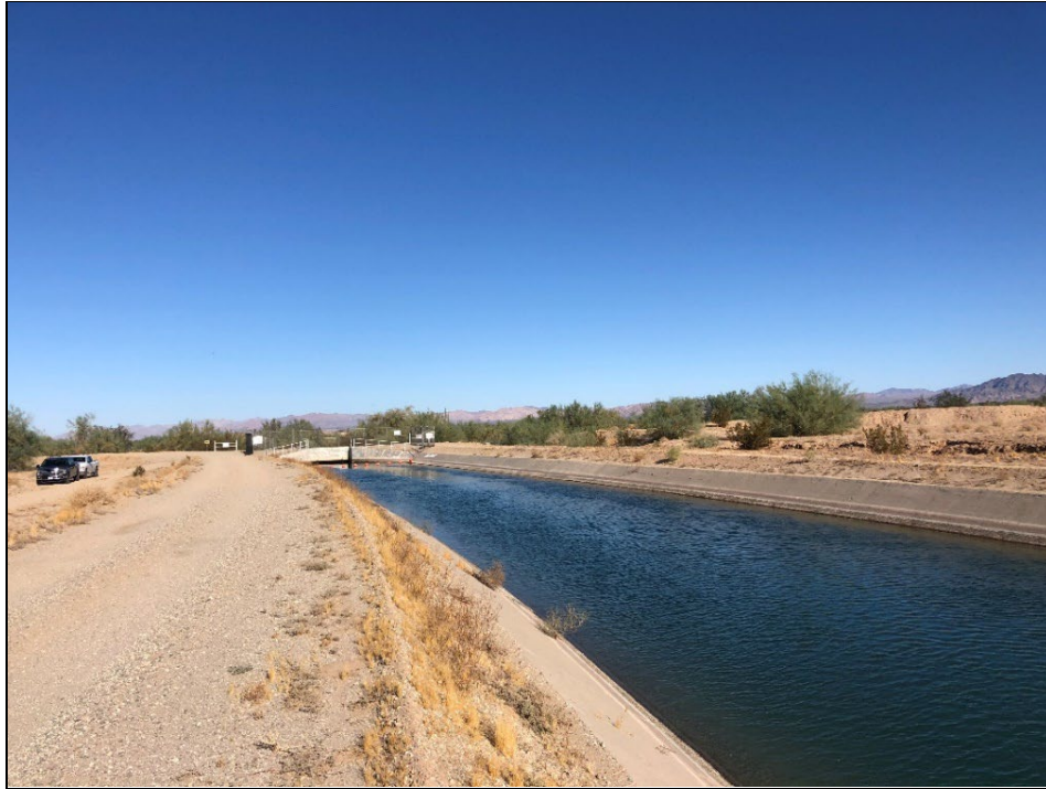
Photo 1. Section of the Coachella Canal adjacent to the Impact Area of Study Area 2; photo facing northwest. November 9, 2020.
