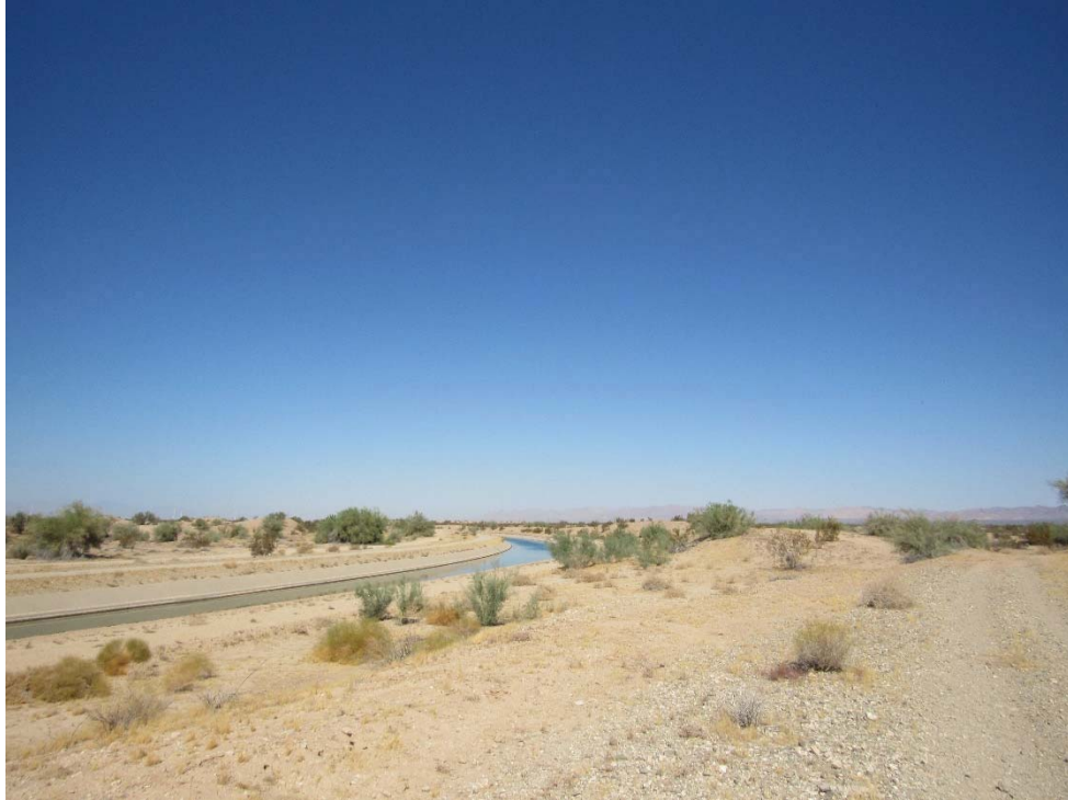
Photo 16: Looking northwest along the east side of the Coachella Canal from the southern boundary of the subject site.
