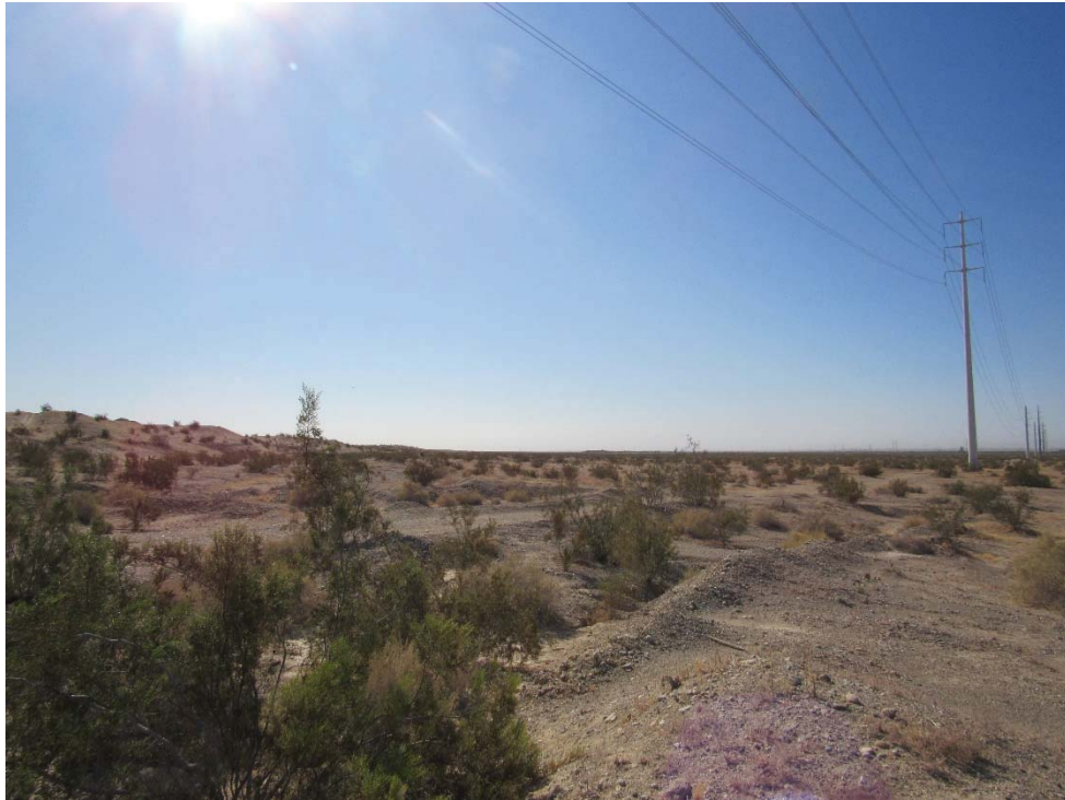
Photo 1: Looking south from the northwest corner of the Clark portion of the subject site at Noffsinger Road and the IID 230kv KN&KS power line.
