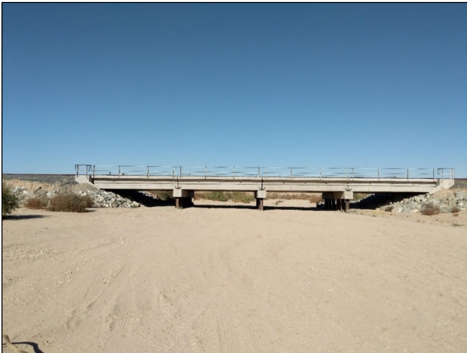
Photo 2. View of the railroad right-of-way within the northeast portion of the Project Area. ED-3001 drainage crosses the railroad via an underpass; photo facing northeast. November 11, 2020.
