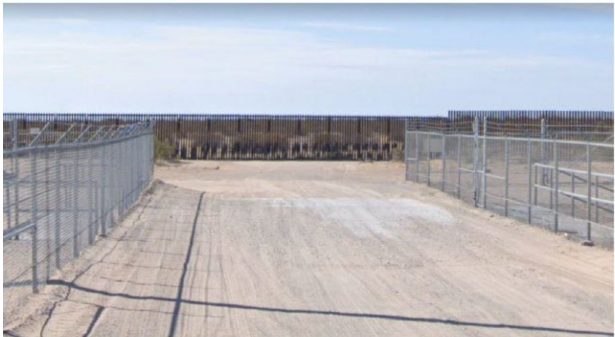
Bridge over south American Canal
