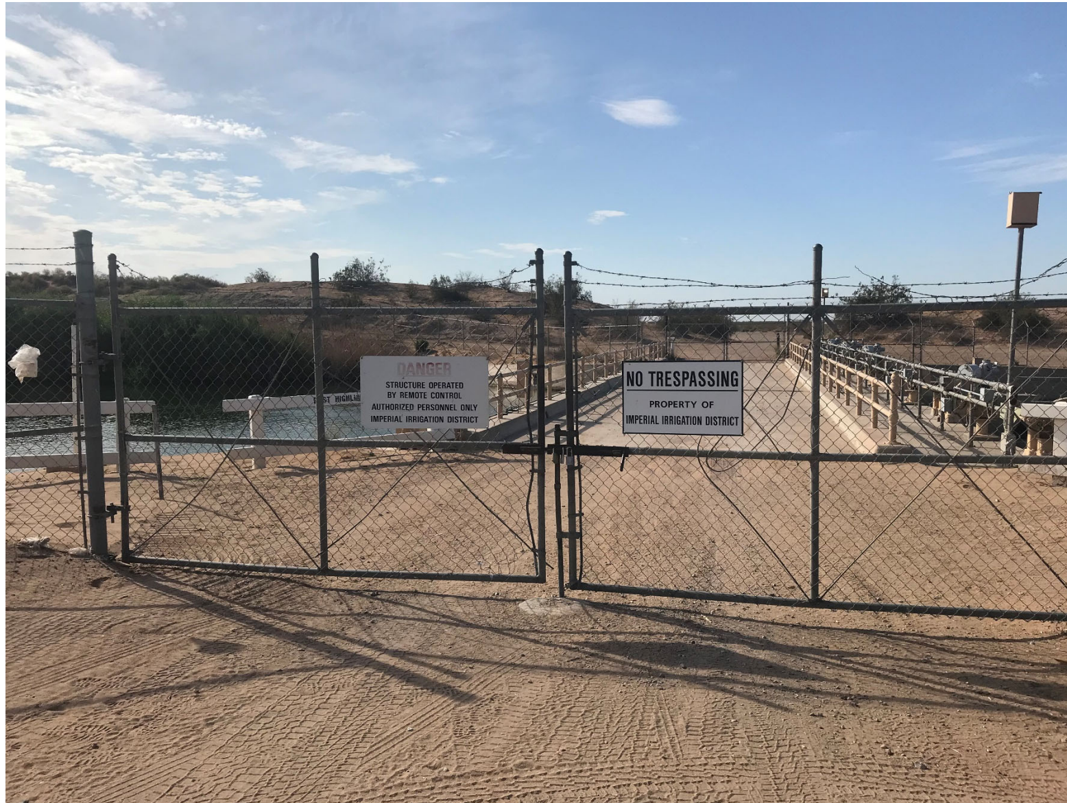
Figure 2-5. Bridge Crossing – Pedestrian Access Only
