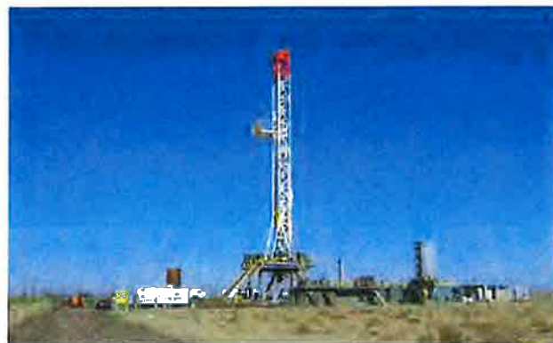
Exhibit 1 – Picture of Example Drill Rig
