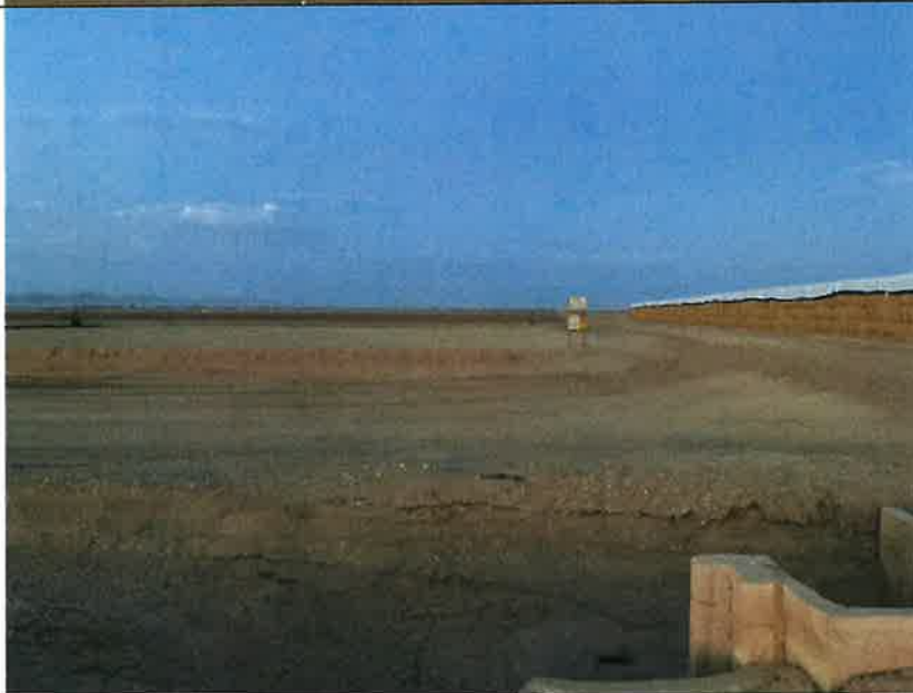
Photo # 5 Orita Well Pad #2
