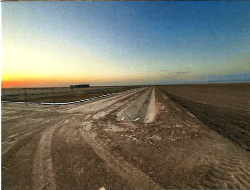
Photo # 3 Dry irrigation ditch
