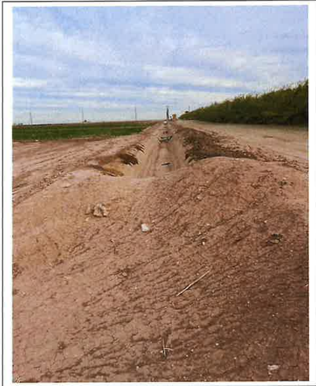
5. Concrete lined ditch facing north from Kemp road facing north
