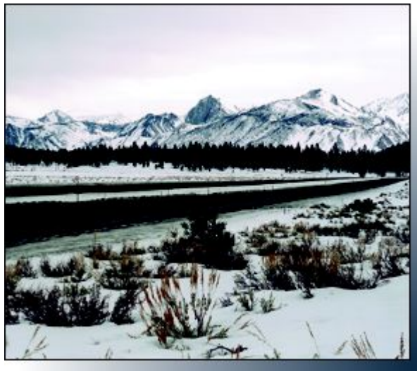
Highway 395, Mono County
