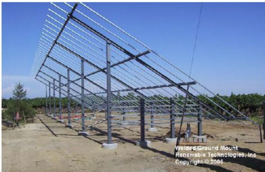
Typical Fixed-Tilt Mounting Structure
