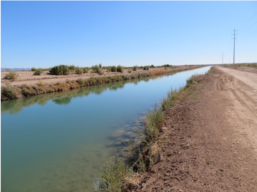
Photo 1: Southeast-facing view of the East Highline Canal along the east side of the project site.
