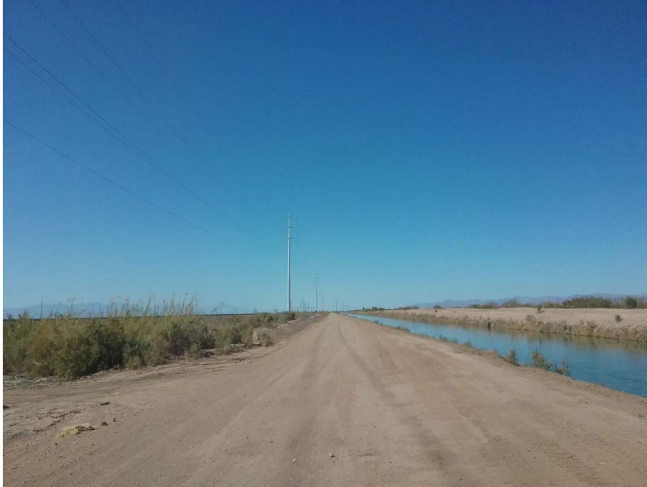
Photo 13: Looking northwest along the IID's East Highline Canal that forms the boundary for the subject sites.
