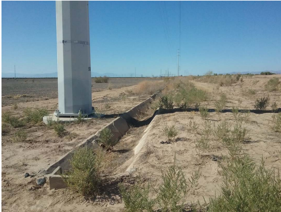
Photo 17: Looking at the concrete lined ditch that runs along the boundary of the southern parcel.
