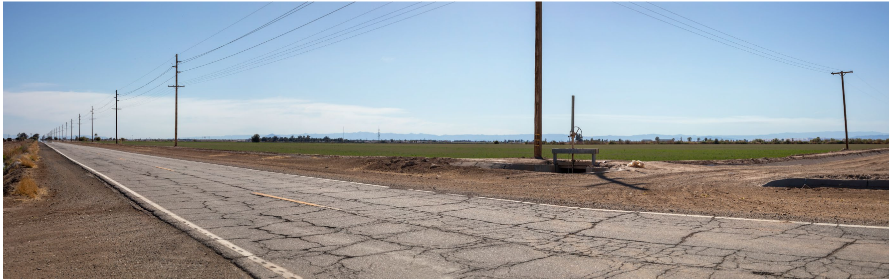
Figure 3.2-2. Existing Key Observation Point 1
