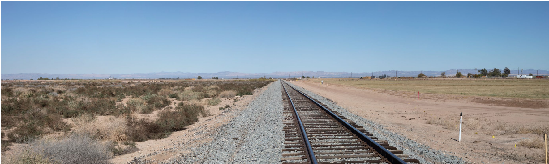
Figure 3.2-4. Existing Key Observation Point 3
