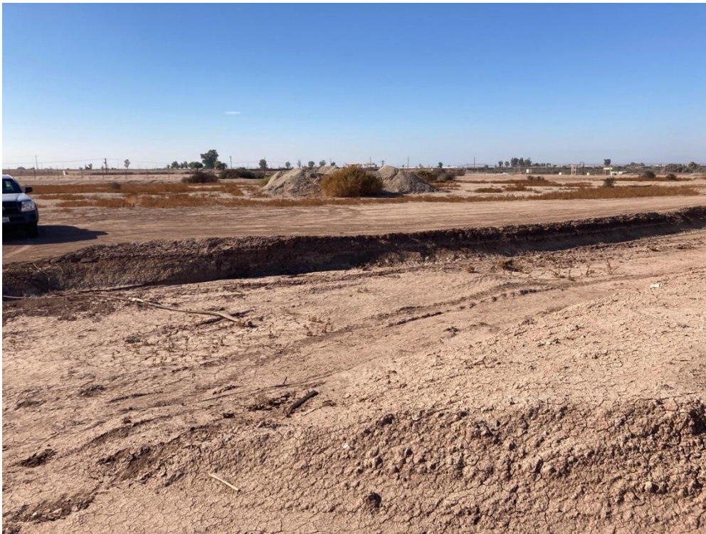
Photo 4. Overview of a man-made ditch leading into a culvert just north of the Livesley Drain. The area above the drainage is a disturbed vegetation community of Cattle Spinach. Photo is facing northwest.
