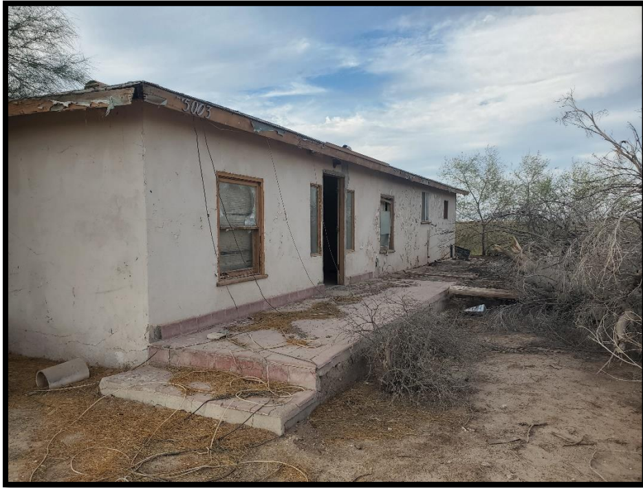
Figure 1: Main residence, facing northwest
