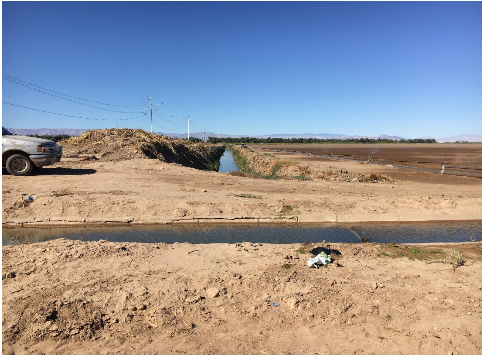
From southwest corner of site, looking west toward Fig Drain No. 1B. Note, concrete lined channel in the foreground is a head ditch that periodically conveys flow for irrigation – a non-jurisdictional drainage.
