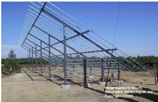
Typical Fixed-Tilt Mounting Structure
