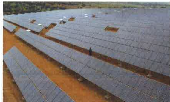
Typical Fixed-Tilt Solar Panel Rows
