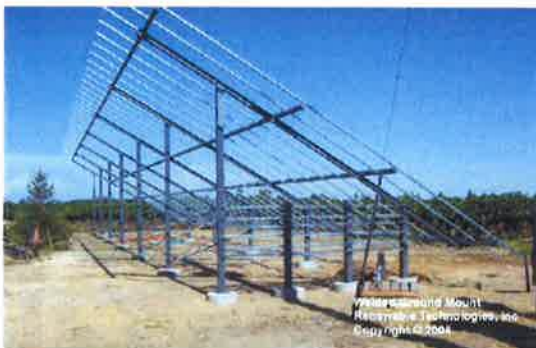
Typical Fixed-Tilt Mounting Structure
