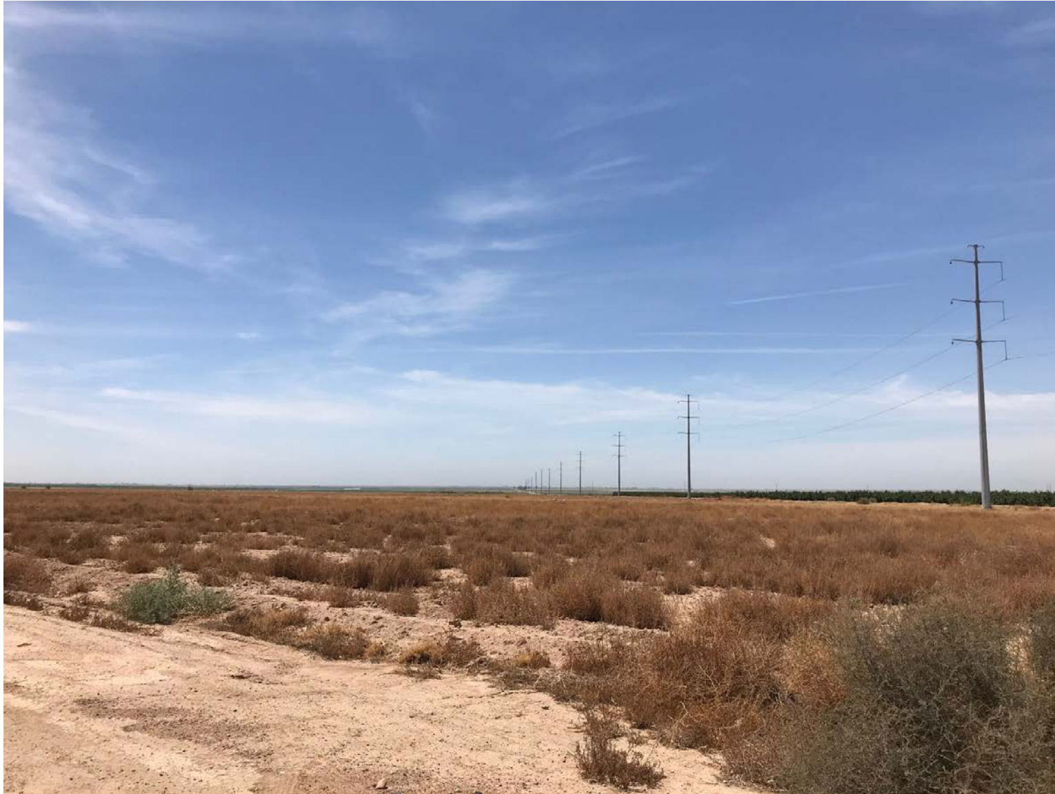
Existing View at Key Observation Point 3
