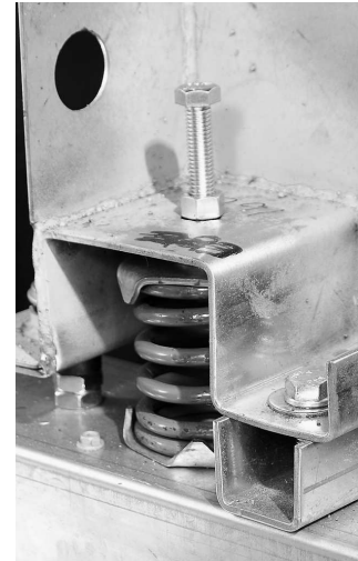
Figure 6. Spring isolation
