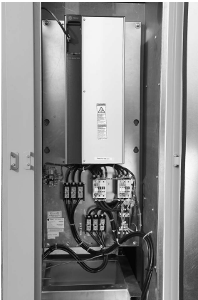
Figure 7. Variable frequency drive
