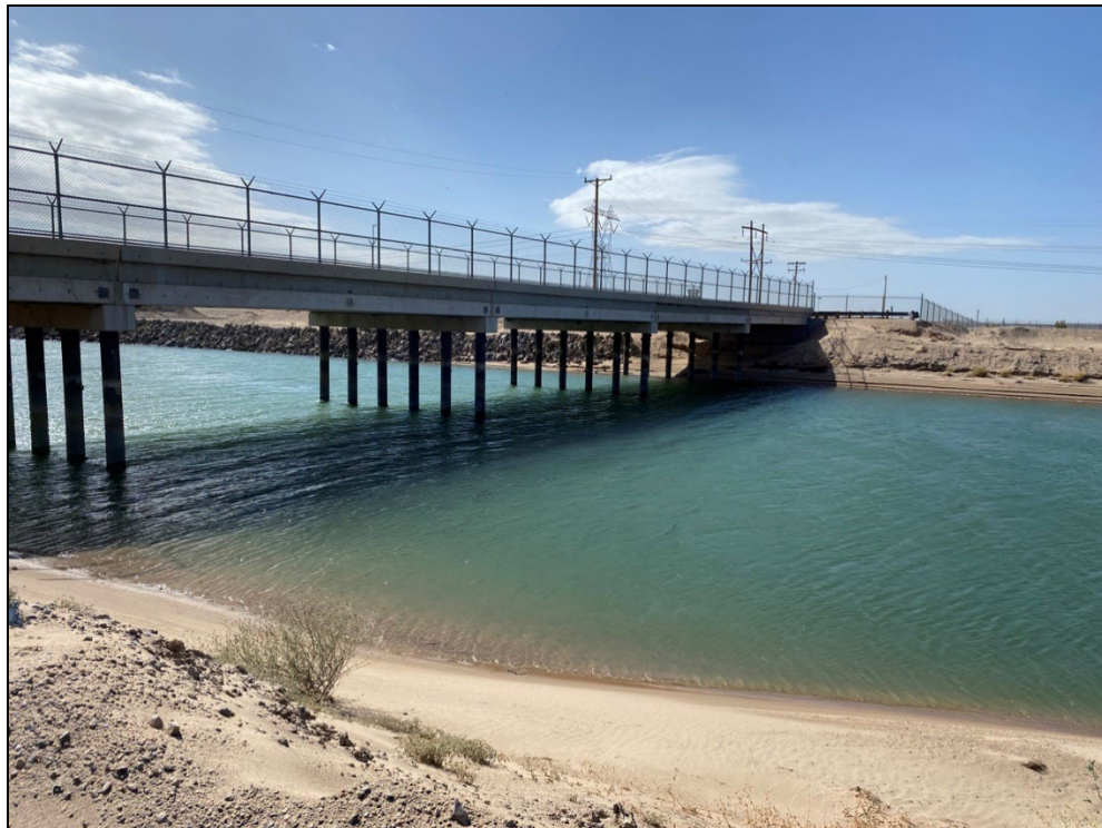
Photo 11. View of the Off-line Storage Canal as it flows beneath the access road bridge in the eastern portion of the Study Area. Photo taken facing southeast. April 12, 2022.
