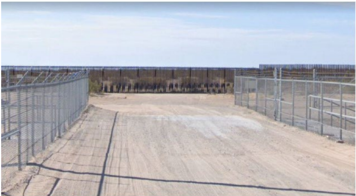
Bridge over south American Canal
