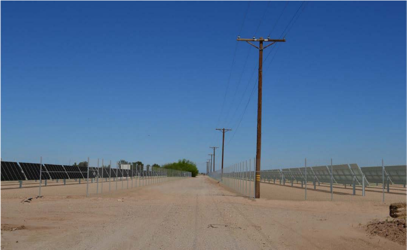
Figure 4.1-5. Key Observation Point 1 – Project View Simulation (Photovoltaic Modules Mounted on Horizontal Single-Axis Tracker System)
