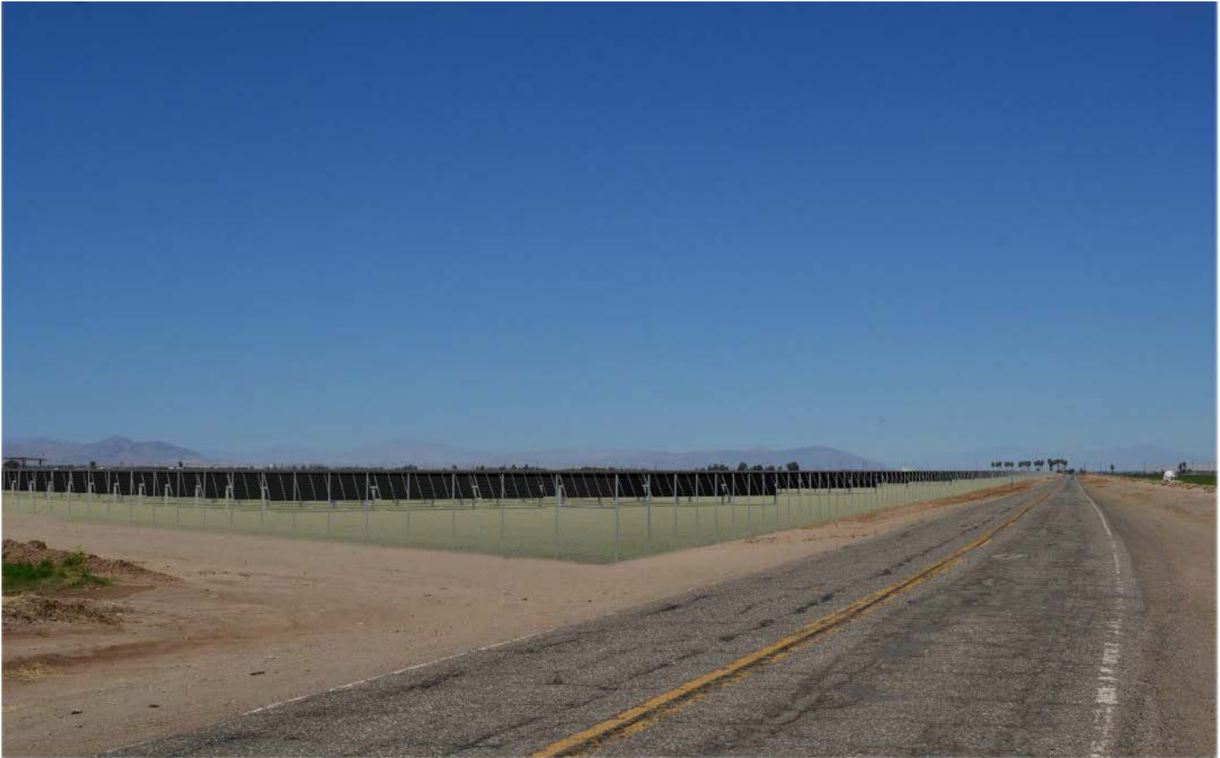
Figure 4.1-8. Key Observation Point 2 – Project View Simulation (Photovoltaic Modules Mounted on Horizontal Single-Axis Tracker System)
