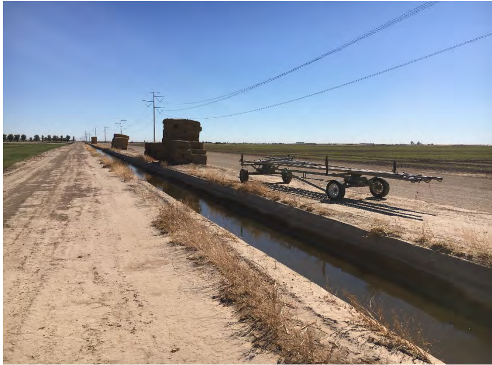
Wormwood Lateral canal – generally carries water year round and would be considered a jurisdictional resource.
