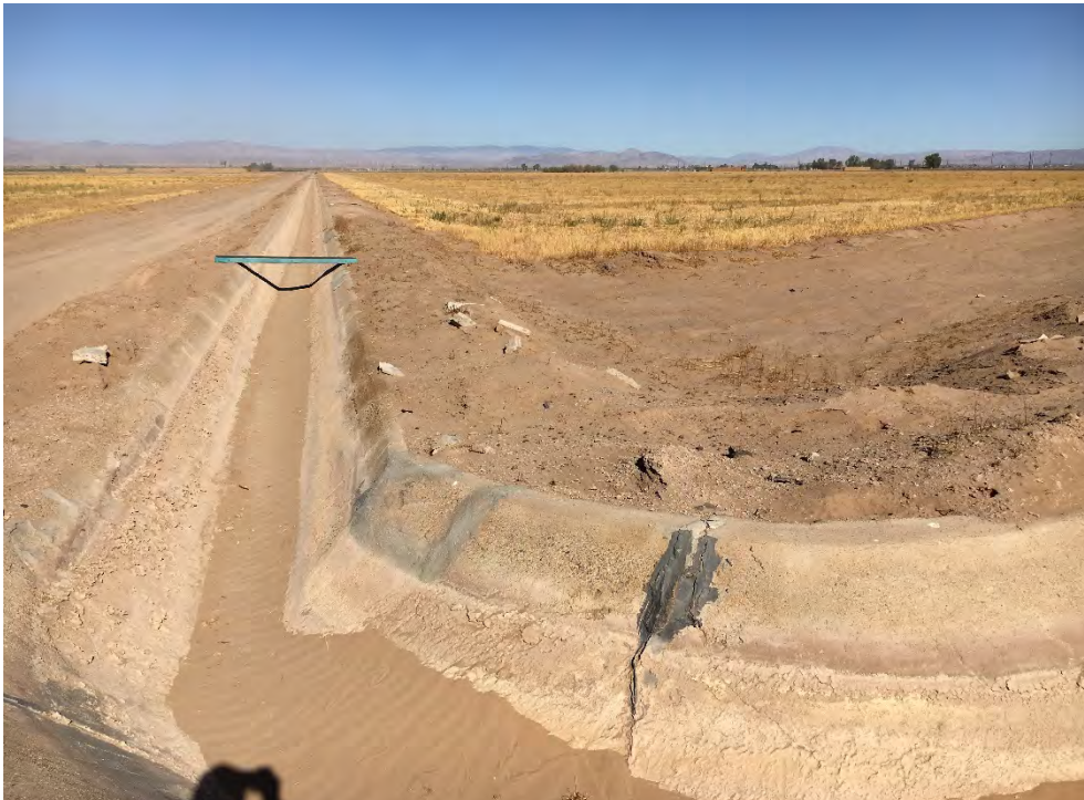
View of central portion of proposed Project site, looking northeast.
