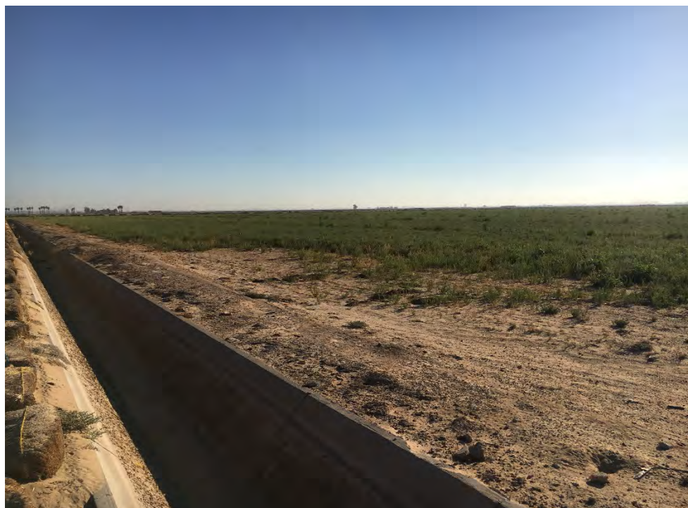
Representative photo of non-jurisdictional irrigation infrastructure.
