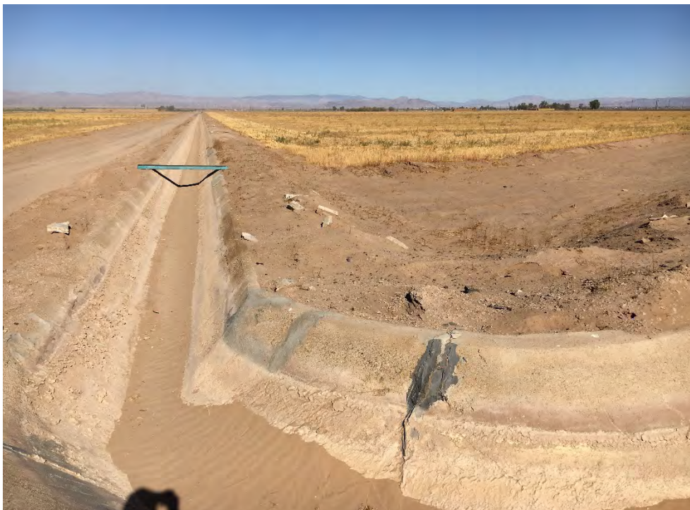
Representative photo of non-jurisdictional irrigation infrastructure.
