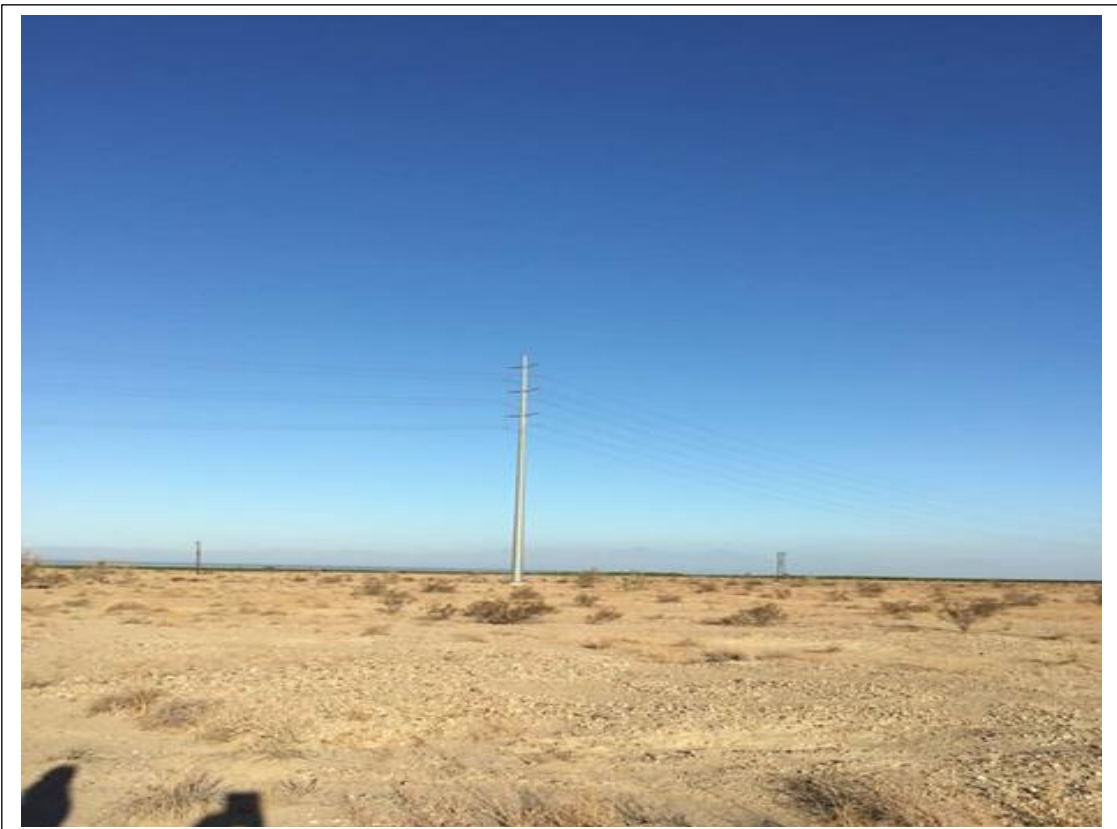
4. Northwest corner facing west; gravelly sand with disturbed soil
