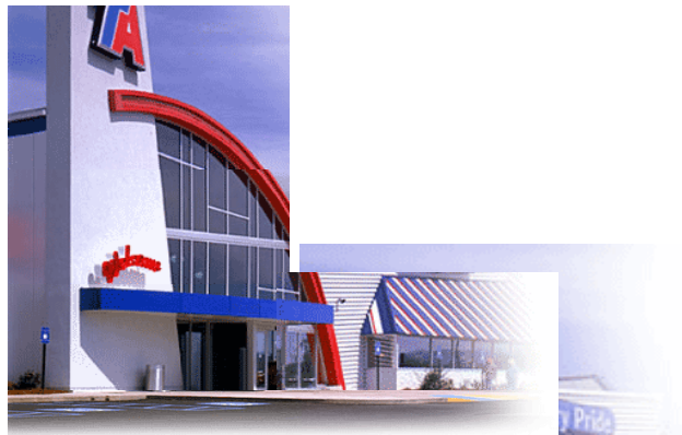
Figure 6 - C Convenience Store & Gas Station
