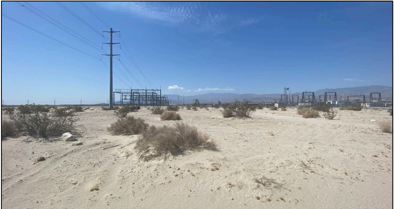
Photo 1: View of the project footprint looking south towards existing Ramon Substation, showing disturbed Creosote Bush Scrub habitat.
