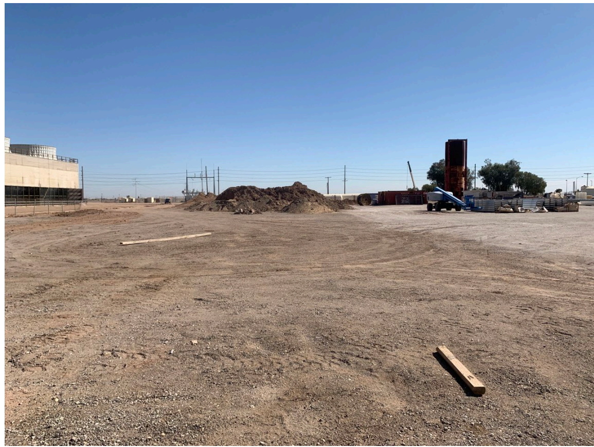
Photo 1: Proposed geothermal energy facilities area located within the existing fenceline, looking east toward Dogwood Rd.
