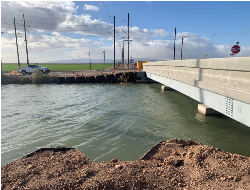
Photo 17: Central Main Canal looking south toward proposed solar energy facility fields. Dogwood Road crosses the Central Main Canal on the right side of the photo. Existing transmission lines currently span the canal.
