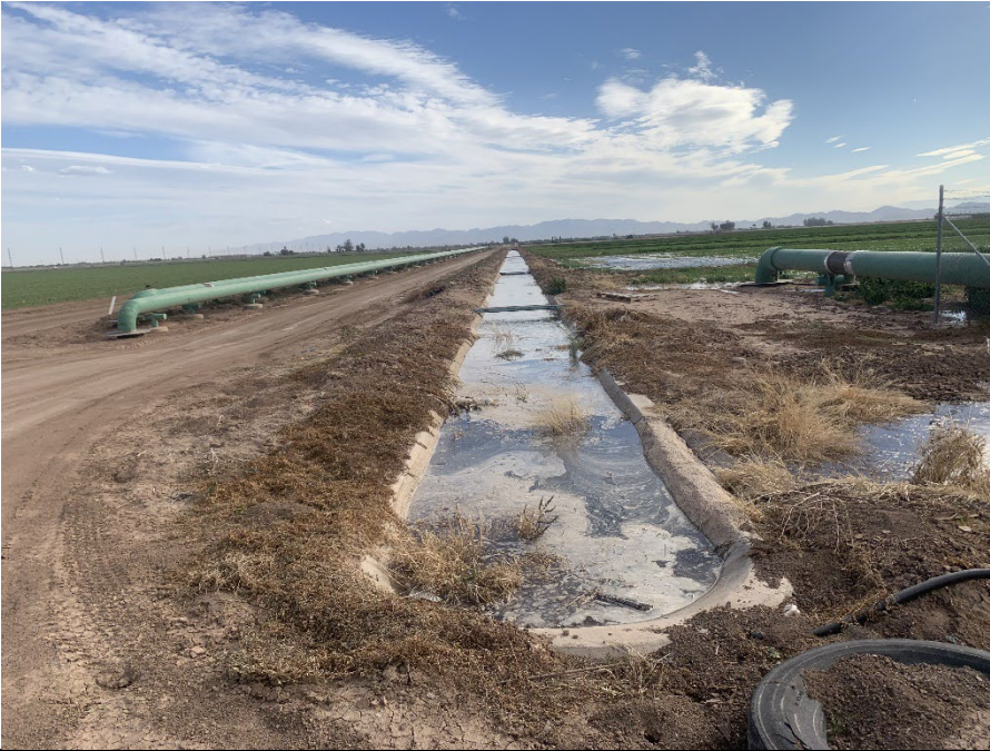
Photo 21: Concrete-lined v-ditch and existing pipeline, looking south. Proposed transmission line would be mounted to the green pipeline on the left side of the frame. Wading birds congregated in the irrigated field on the right (west) field during site visit in February 2023.
