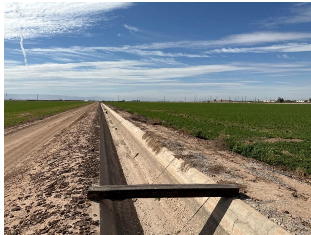
Photo 5: New pipeline alignment, showing the middle of the proposed solar field with agricultural fields (alfalfa) on both sides and lined canal through the middle, looking west.
