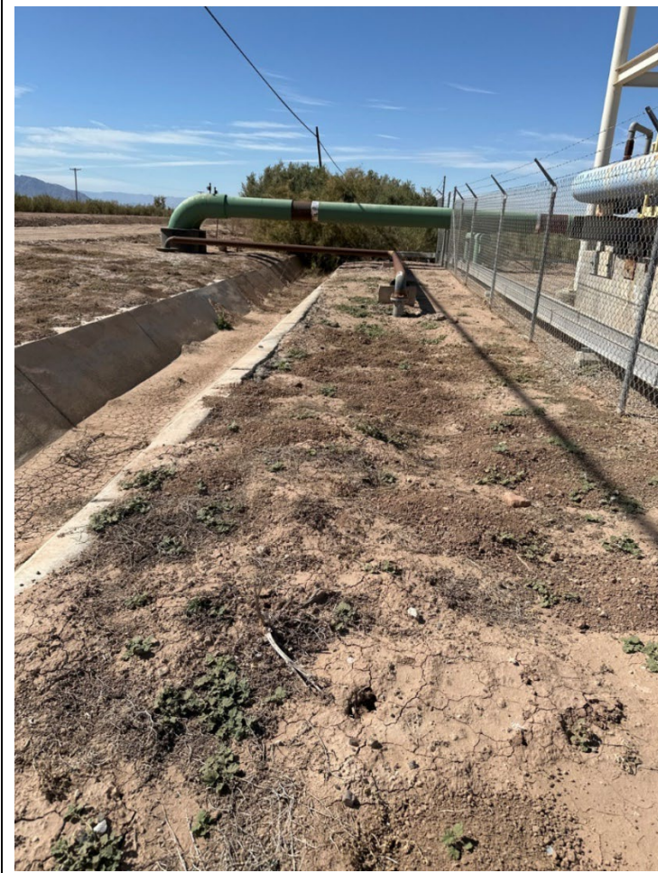
Photo 15: Existing pipeline location south of the geothermal site and adjacent to existing solar field, looking west. Old drainage ditch is shown on the left. Transmission line would span the road and canals/drains aerially, then rejoin the existing pipeline using trays.
