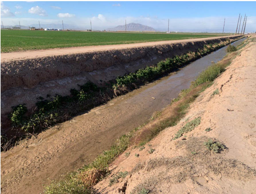
Photo 8: Beech Drain looking west.
