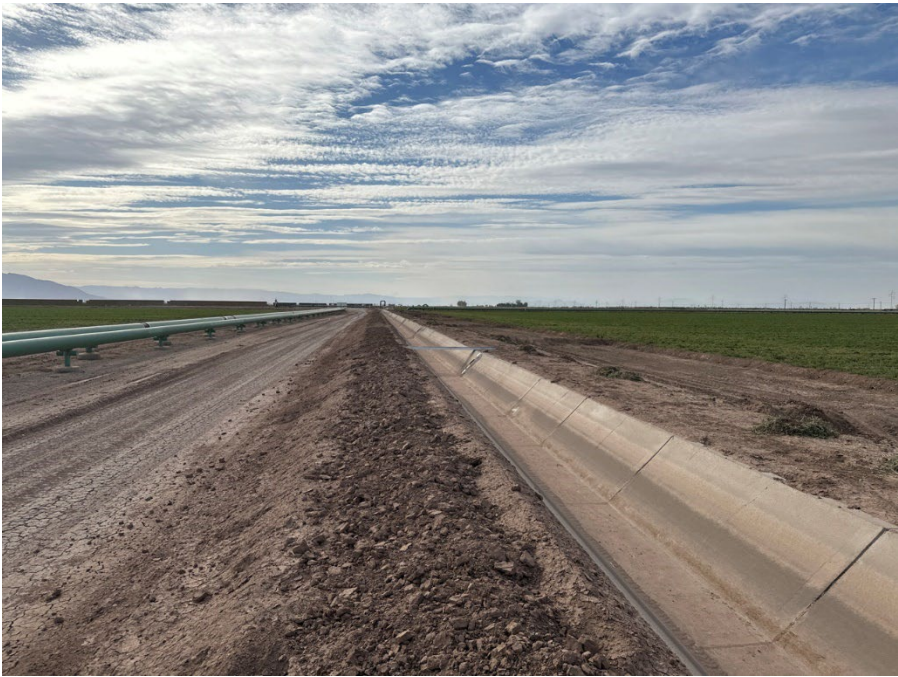
Photo 11: Pipeline and existing canal west of proposed solar field and west of Dogwood Road, looking west.
