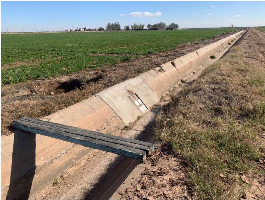
Photo 9: Solar field canal looking east.
