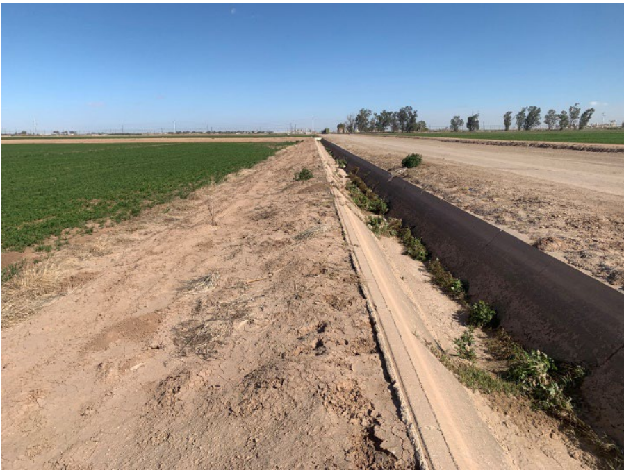
Photo 10: Solar field canal looking north.
