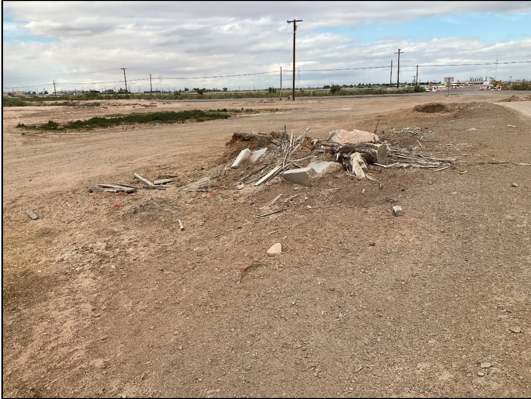
Figure 5-5. Construction debris at the northeast corner of the Dogwood Parasitic Solar Energy Facility site, facing west
