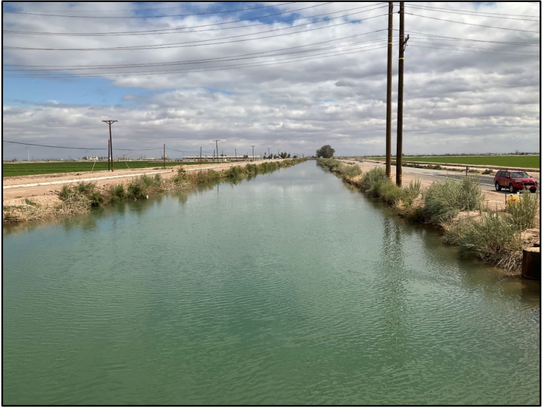
Figure 5-8. CM Canal from Dogwood Road Bridge, facing east
