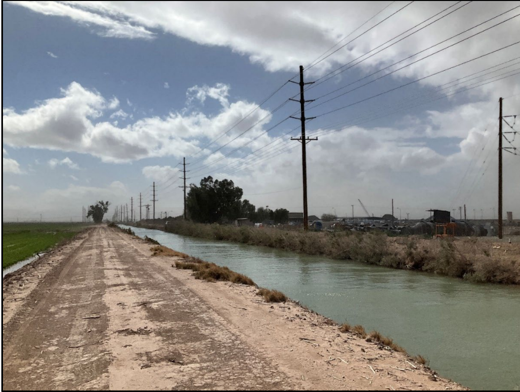
Figure 5-10. Portion of Dogwood Canal located west of Dogwood Road, facing south
