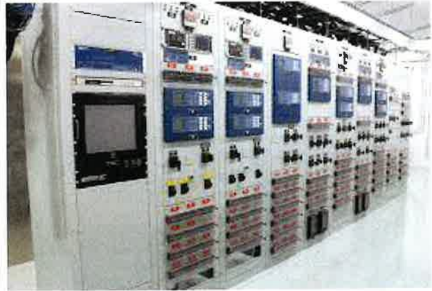
The substation will include a small unmaned control house to house monitoring and protection equipment
