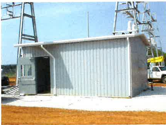
The substation will include a small unmaned control house to house monitoring and protection equipment
