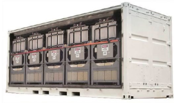
Figure 2-8. Representative Example of Battery Energy Storage Systems
