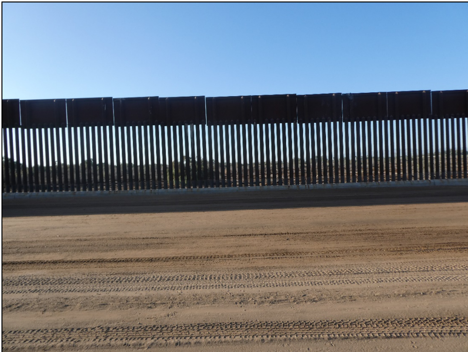
Photo 10. View of border wall lining the southern perimeter, facing south.
