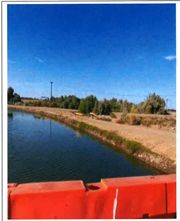
5. Facing south while on bridge 8/8
