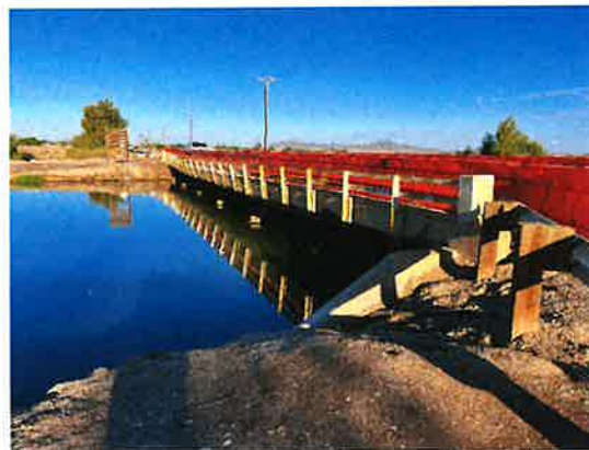
Figure 8: South side of the Picacho Bridge taken from the eastern end of the bridge, view to the west
