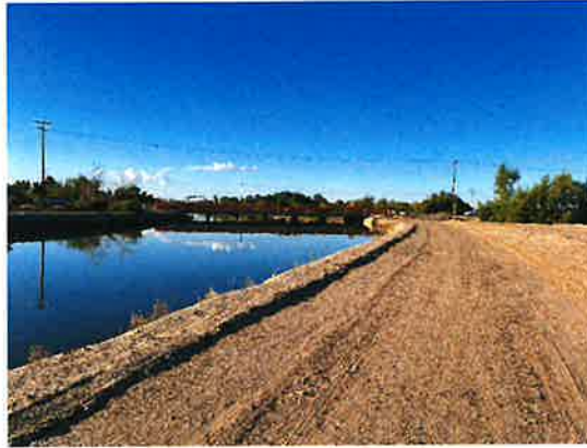
Figure 7: Overview of Yuma Main Canal and Picacho Bridge access road, view to the south-southeast
