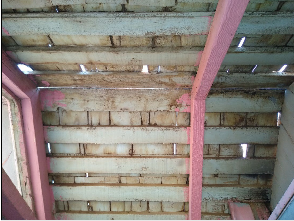
Photo 11: Interior of bat roost outhouse structure.
