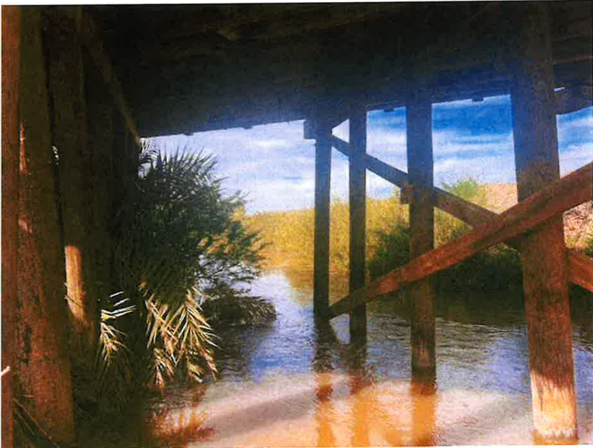
Photograph 8: Detail of the underside of Meloland Bridge. View west, April 2, 2024.
