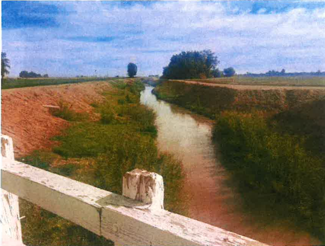
Photograph 3: Overview of the Central Drain Canal as seen from the Meloland Bridge. View west, April 2, 2024.
