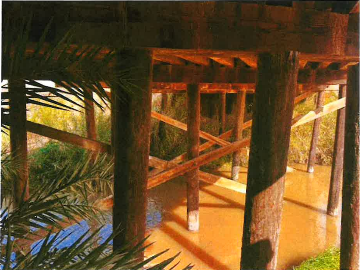
Photograph 7: Detail of the underside of Meloland Bridge. View north, April 2, 2024.
