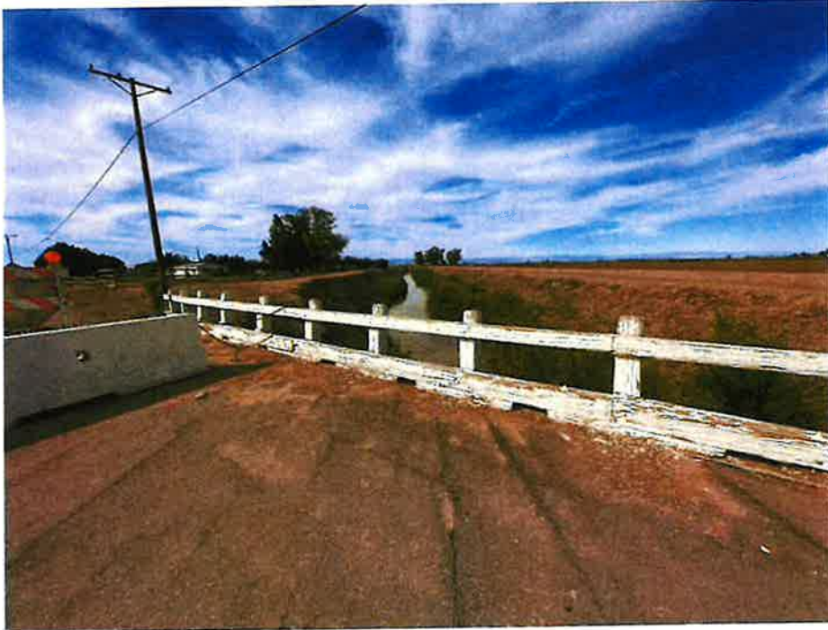
Photograph 5: Southwest-facing view from Meloland Bridge.
