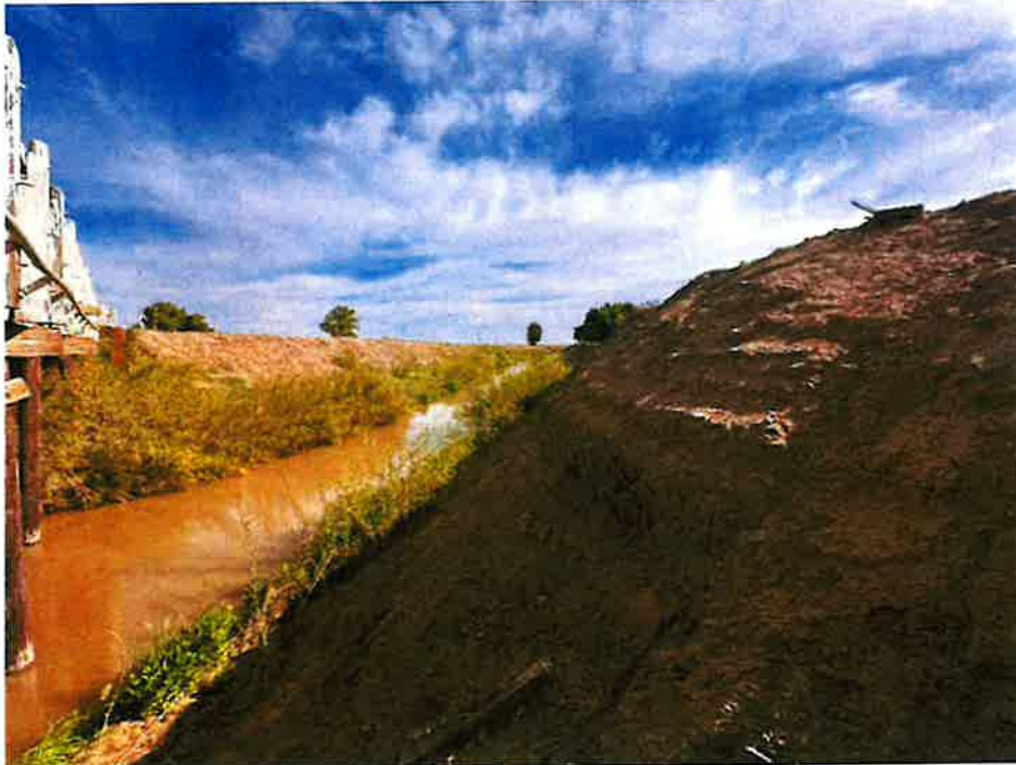
Photograph 2. Northeast-facing view from under the east side of Meloland Bridge.
