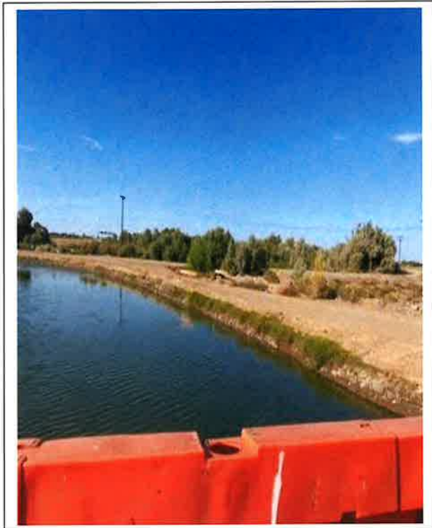
5. Facing south while on bridge 8/8
