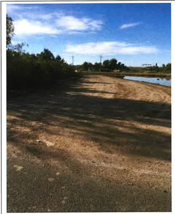
1. The east bank south of Picacho Road. was surveyed
