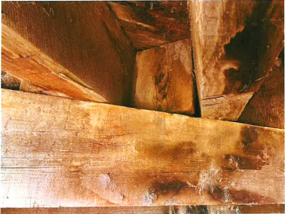
Photograph 9: Detail of the underside of Meloland Bridge. Looking up, April 2, 2024.
