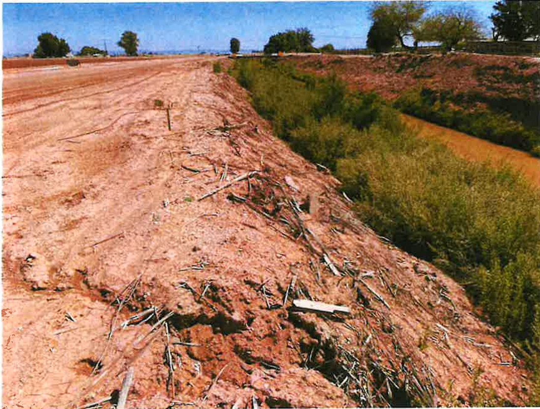
Photograph 5: North side of the Central Drain Canal. View northeast, April 2, 2024.
