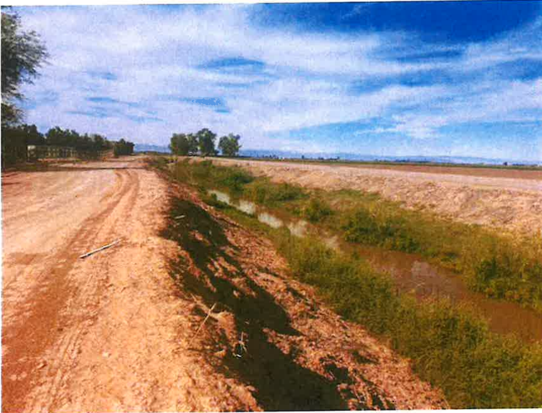
Photograph 2: Overview of the Central Drain Canal. View southeast, April 2, 2024.
