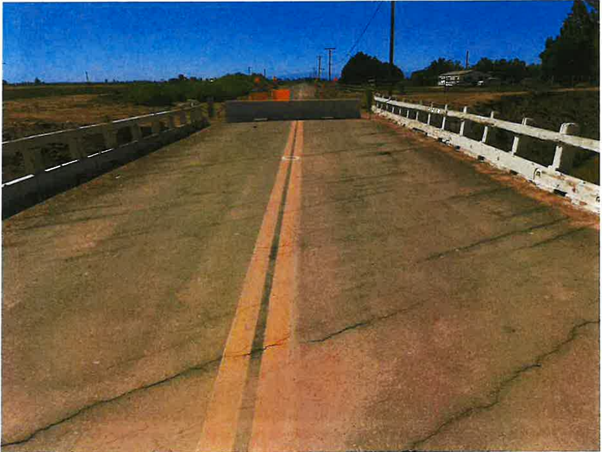
Photograph 5: View of Meloland Road over Meloland Bridge. View north, April 2, 2024.
