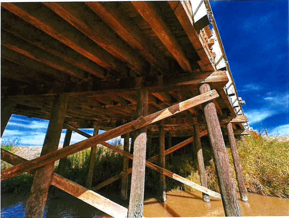
Photograph 6: Detail of the underside of Meloland Bridge. View north, April 2, 2024.
