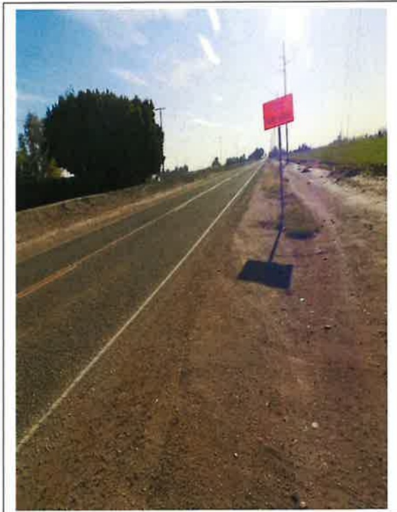
12. Residence, Ross Road to left and site to right; looking east
