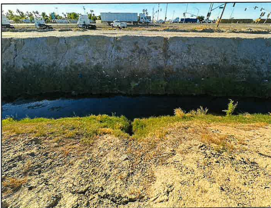
Figure 12. Side wall of Acacia Five A Drain, facing west
