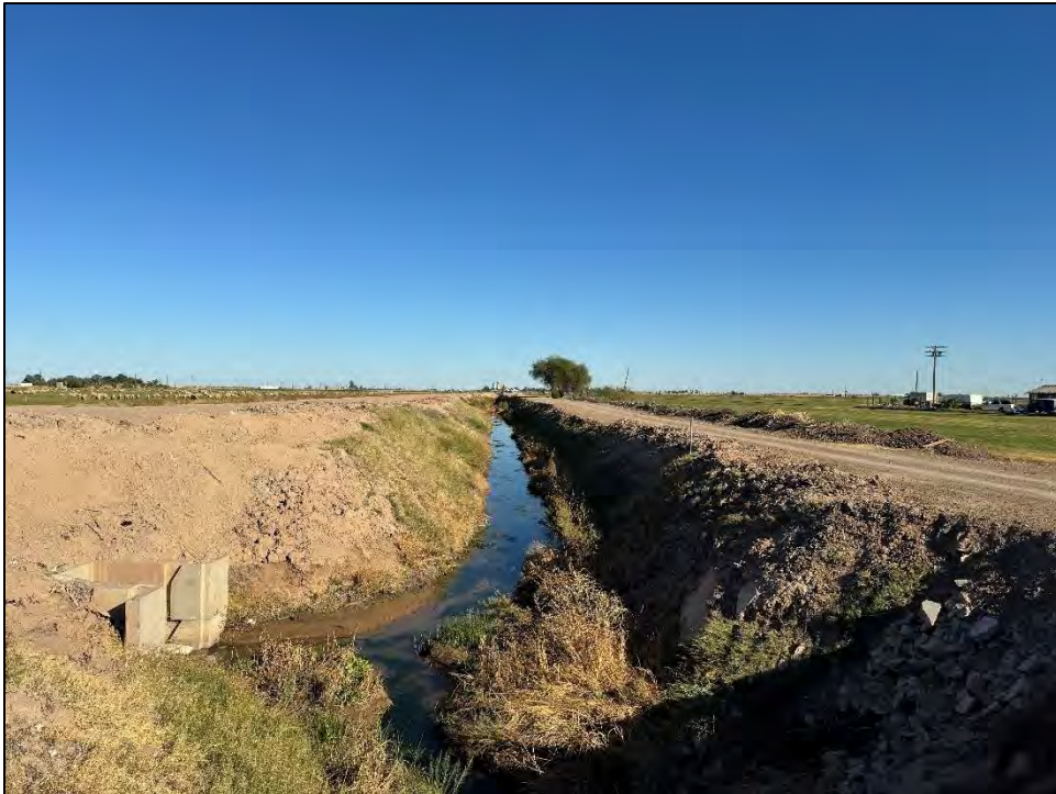
Figure 11. Northern portion of Acacia Five A Drain in Project Area, facing south
