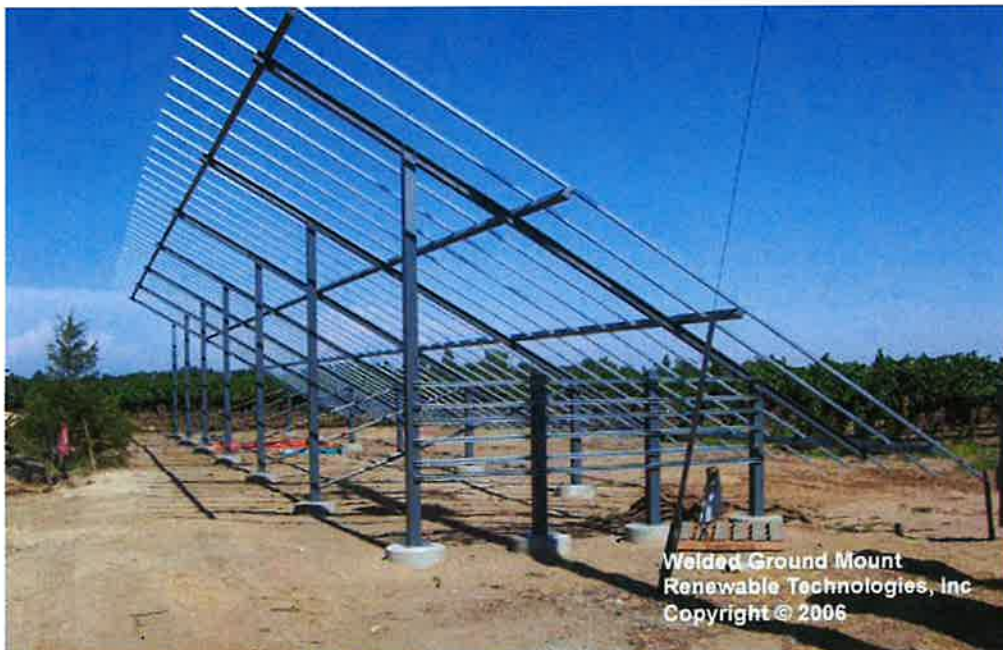
Typical fixed-tilt mounting structure
