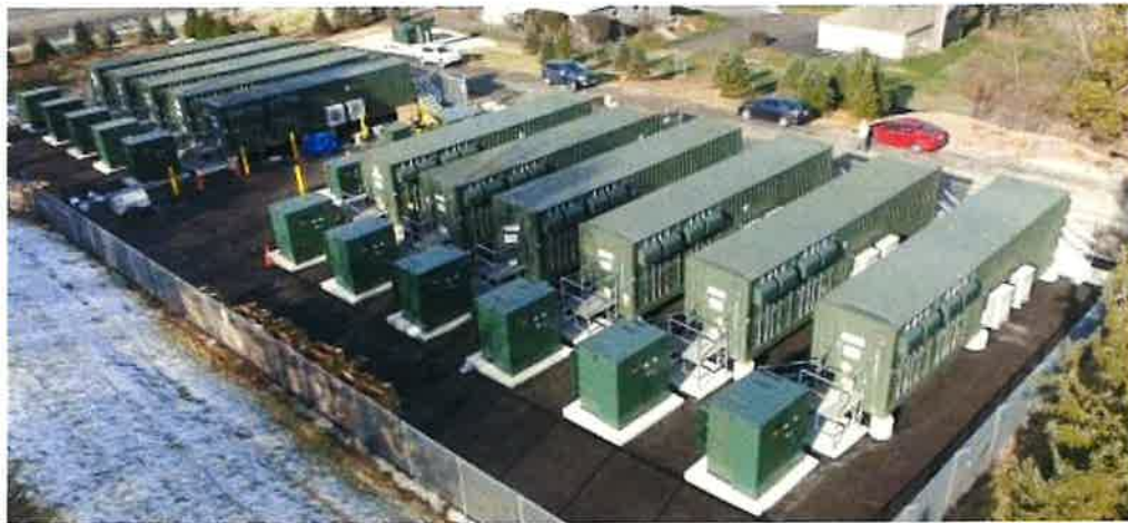
BESS Installed in Dedicated Structure
