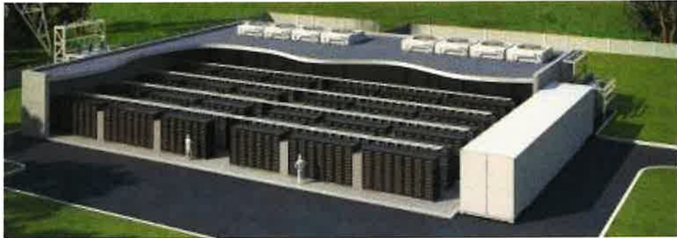
BESS Installed in Dedicated Structure
