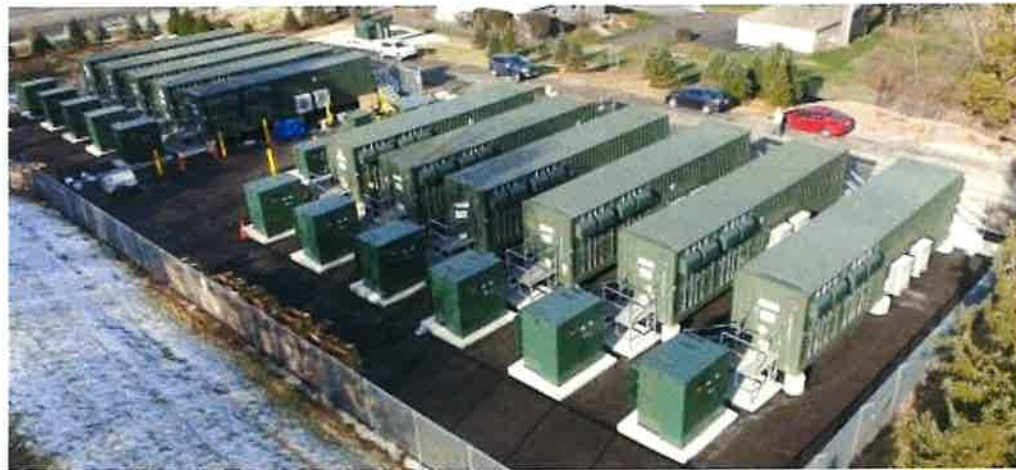
BESS Installed in Dedicated Structure
