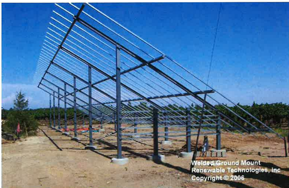
Typical fixed-tilt mounting structure
