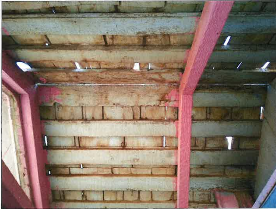
Photo 11: Interior of bat roost outhouse structure.
