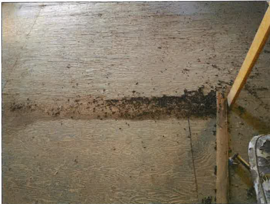
Photo 14: Interior of bat roost building, guano pile on floor.
