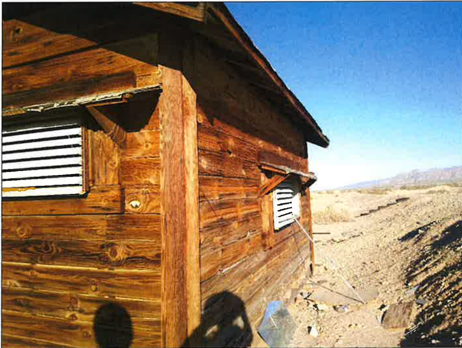
Photo 12: Exterior of bat roost building.
