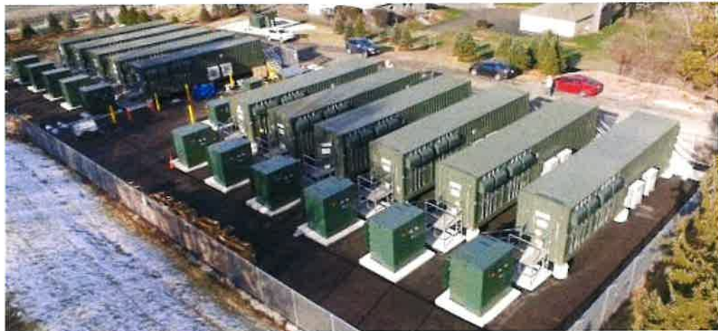
BESS Installed in Dedicated Structure
