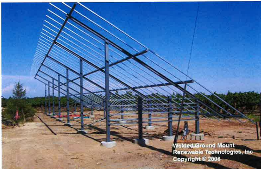
Typical fixed-tilt mounting structure
