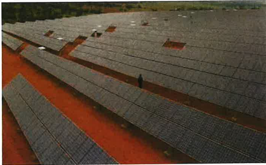
Typical fixed-tilt solar panel rows
