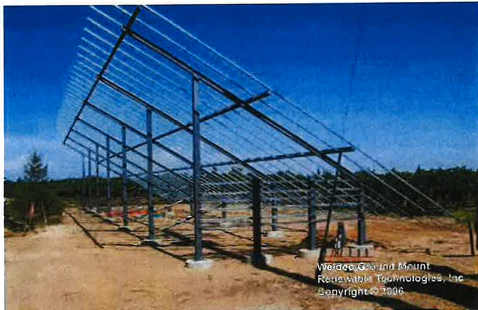
Typical fixed-tilt mounting structure
