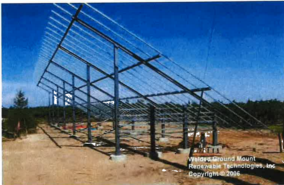
Typical fixed-tilt mounting structure
