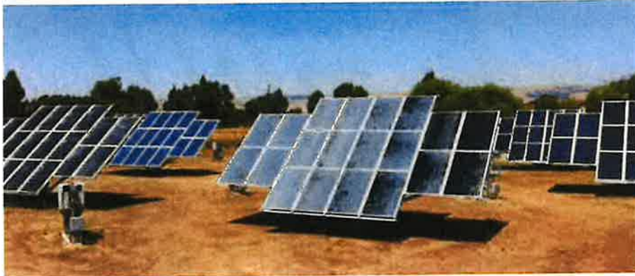
Typical dual axis tracking solar panels
