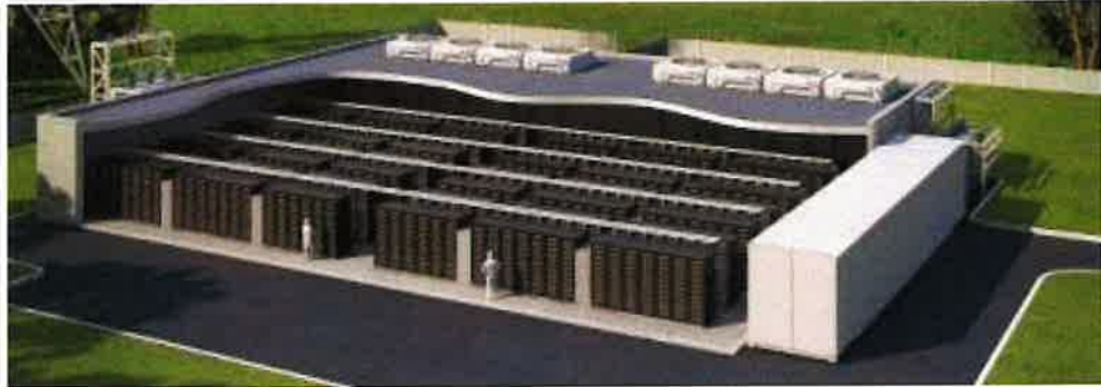
BESS Installed in Dedicated Structure
