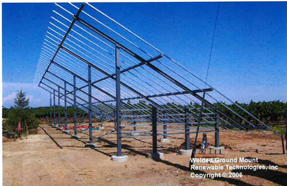
Typical fixed-tilt mounting structure
