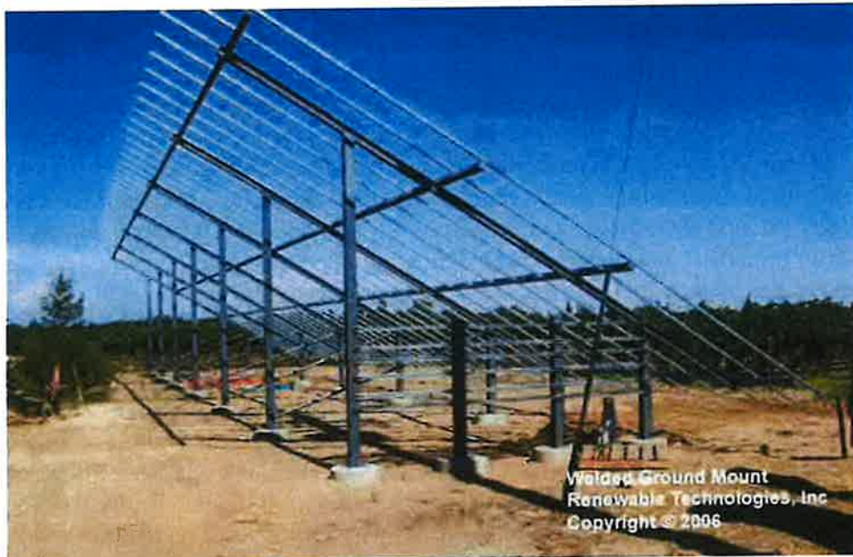
Typical fixed-tilt mounting structure
