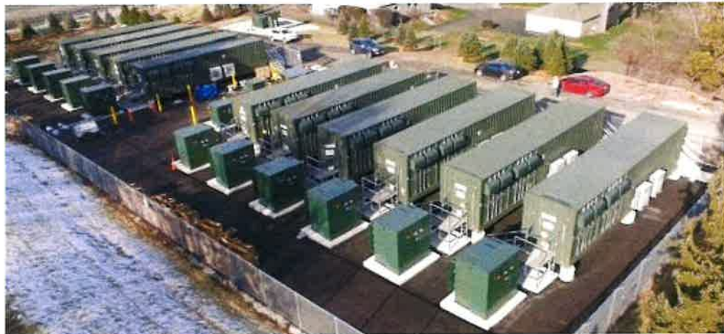
BESS Installed in Dedicated Structure
