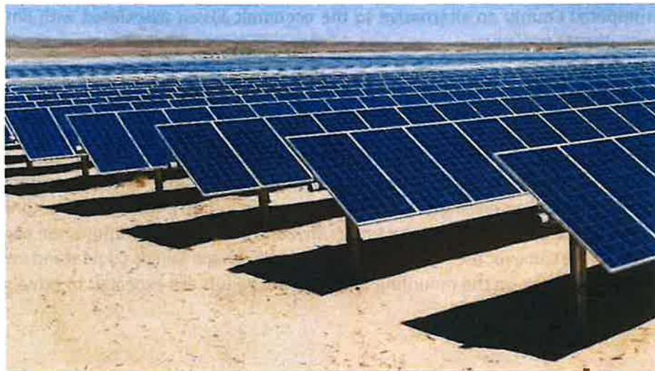
Typical single axis tracking solar panels
