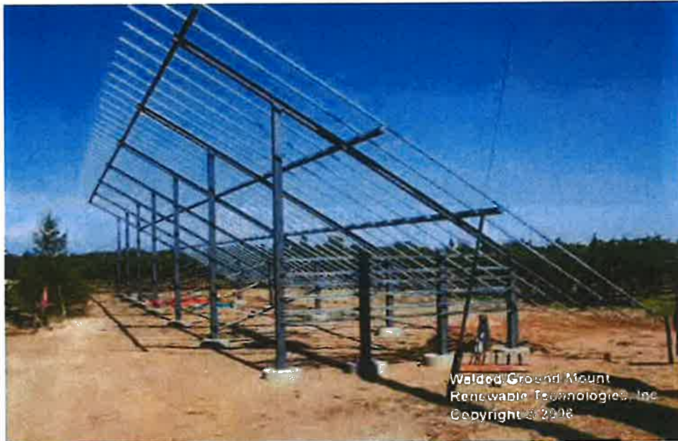
Typical fixed-tilt mounting structure
