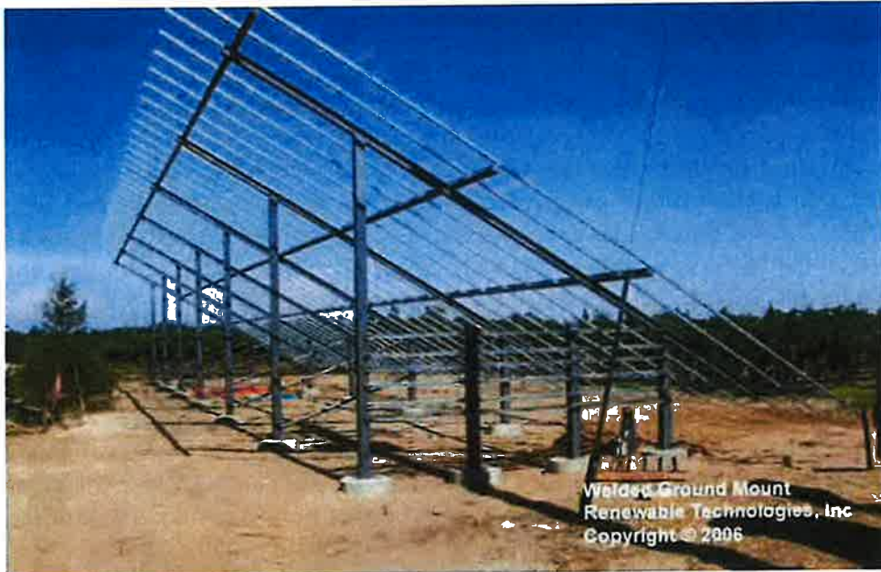
Typical fixed-tilt mounting structure
