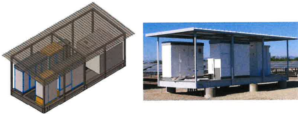
Typical inverter stations
