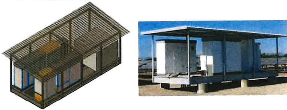
Typical inverter stations
