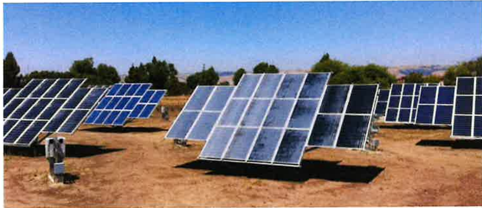
Typical dual axis tracking solar panels
