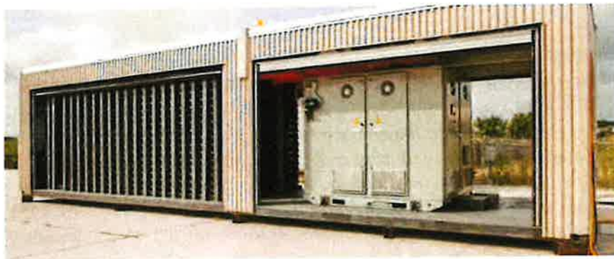
Typical BESS module configuration
